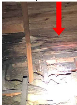
Example of energized knob and tube in contact with insulation. Recommend repair as needed.
