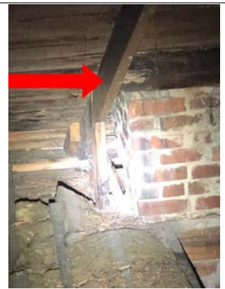
Example of moisture damage at eaves.
