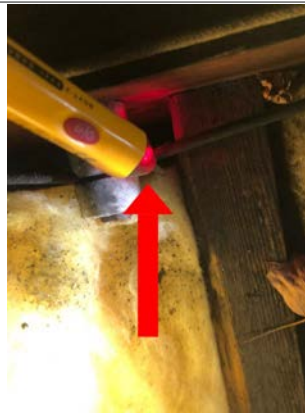
Example of energized knob and tube in contact with insulation. Recommend repair as needed.
