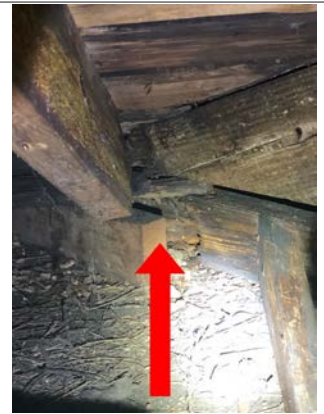
Example of moisture damage at eaves.
