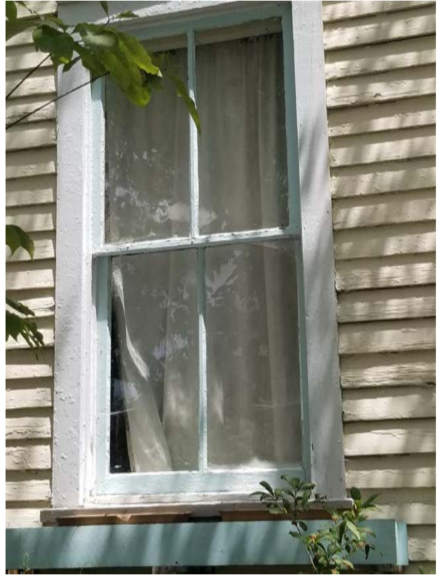
TYPICAL WINDOW TO BE REPLACED
