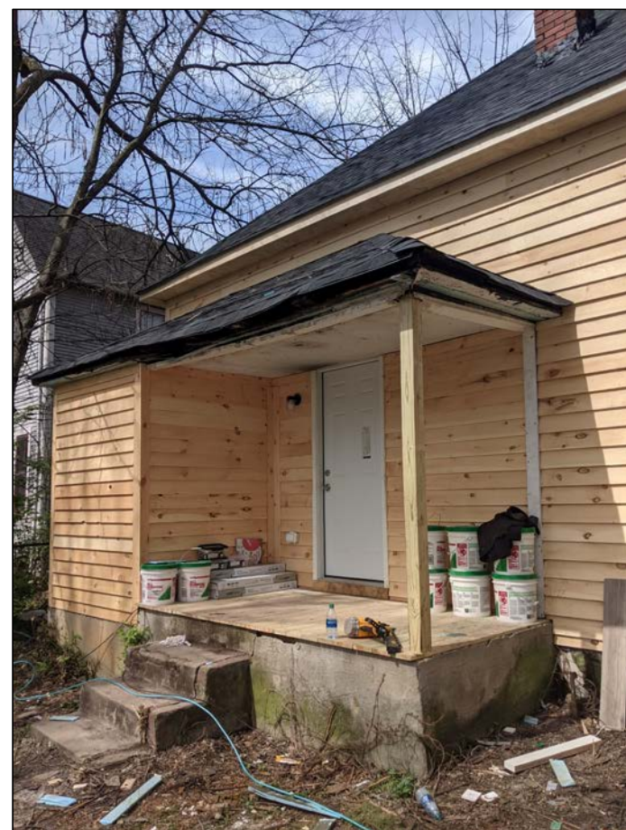
Rear porch modifications; replaced door
