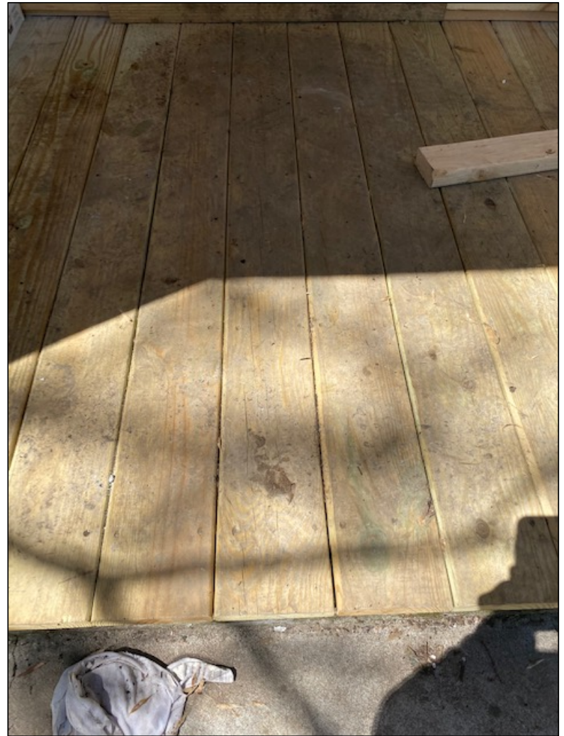
Rear porch decking already installed
