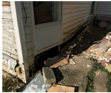
WALL SUPPORTED DIRECTLY ON EARTH
