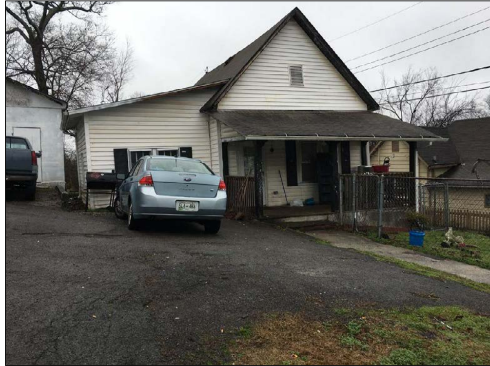
Photo provided by applicant, prior to work
