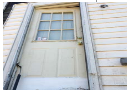
REPLACED ORIGINAL FRONT DOOR
