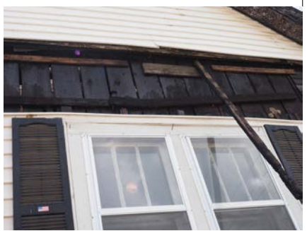
SIDING OVER BURN WOOD PLANKS
