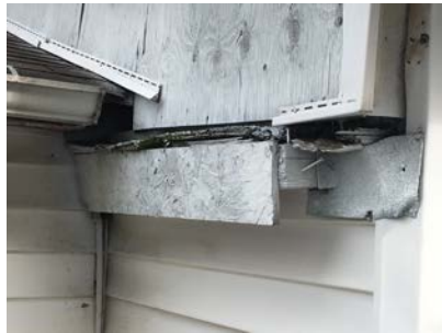
DEFECTIVE CONNECTION AT ADDITION
