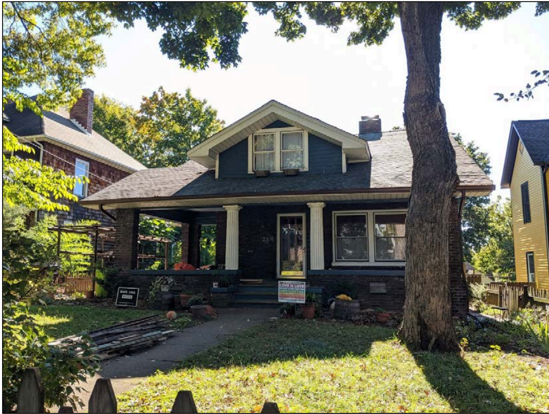
Existing conditions, showing fluted columns and vinyl lap siding on dormer.
