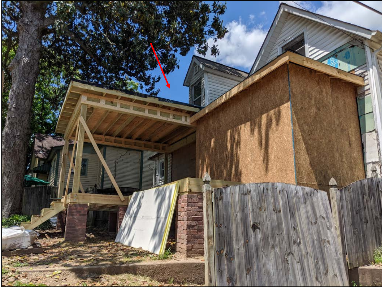
Rear view from alley
