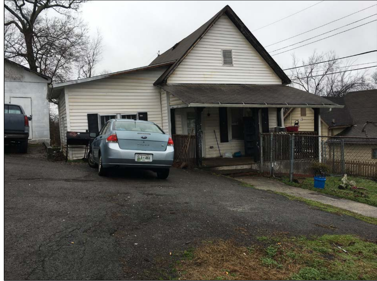
Photo provided by applicant, prior to work
