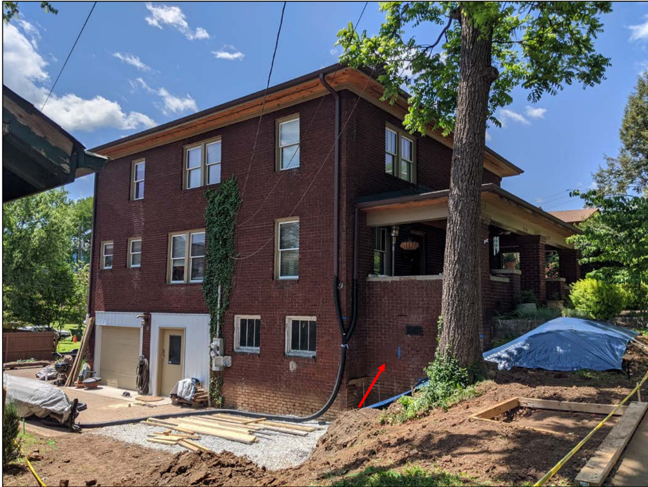
Northeast oblique view: elevation to receive new door and retaining wall
