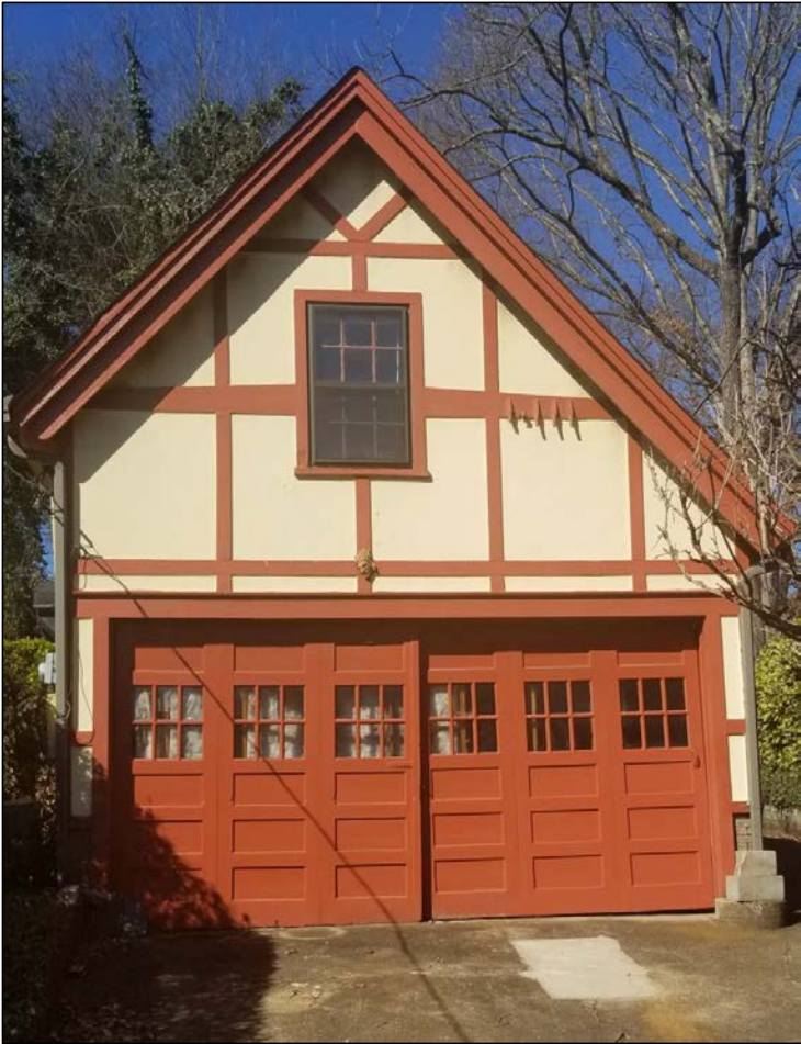
Garage and existing doors
