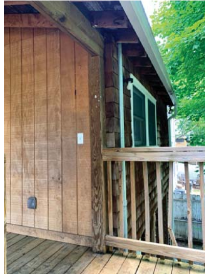
Porch visibility, unoriginal material, and damage. Also visible in left photo, foundation damage.
