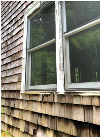
Siding and window damage, unoriginal front door from early 2000's.
