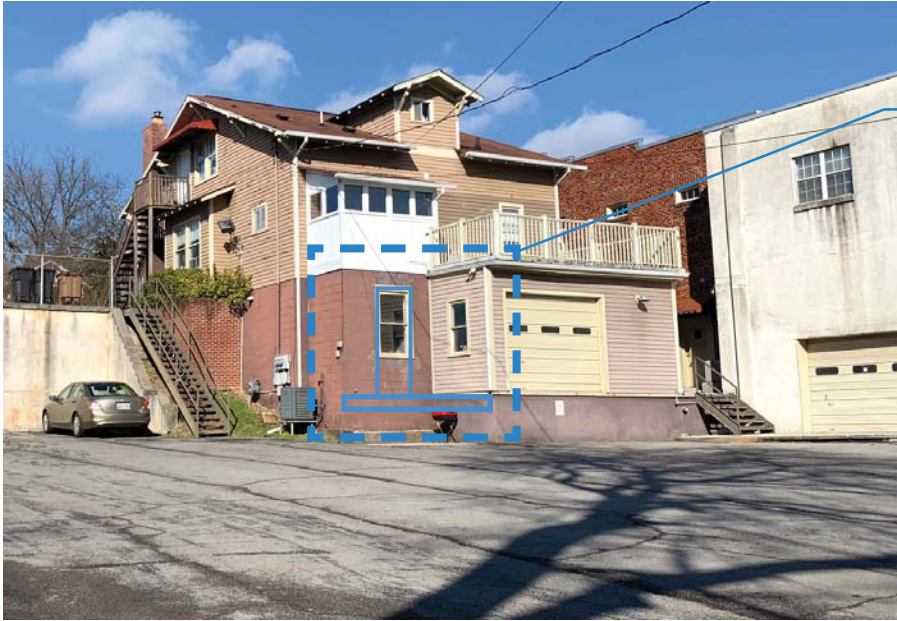
● Location of proposed new door and access platform. This is completely invisible from the street.
