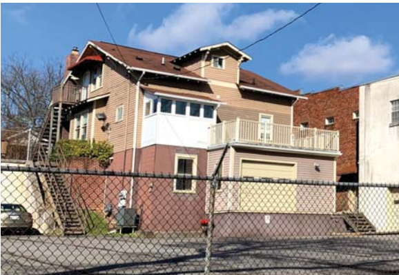
Before - Rear View
