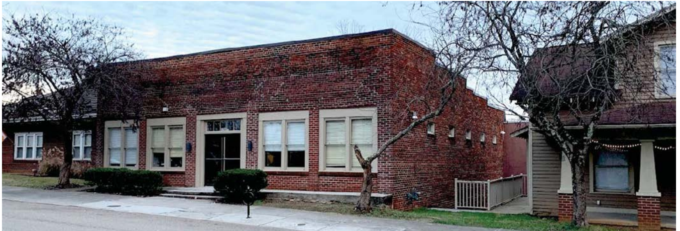
View down West Elevation from Front Elevation, the rear of the building is hidden by adjacent residence
