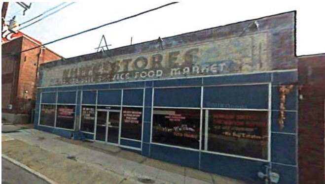
1208 N Central St | 2007 and 2019 (aluminum windows)
