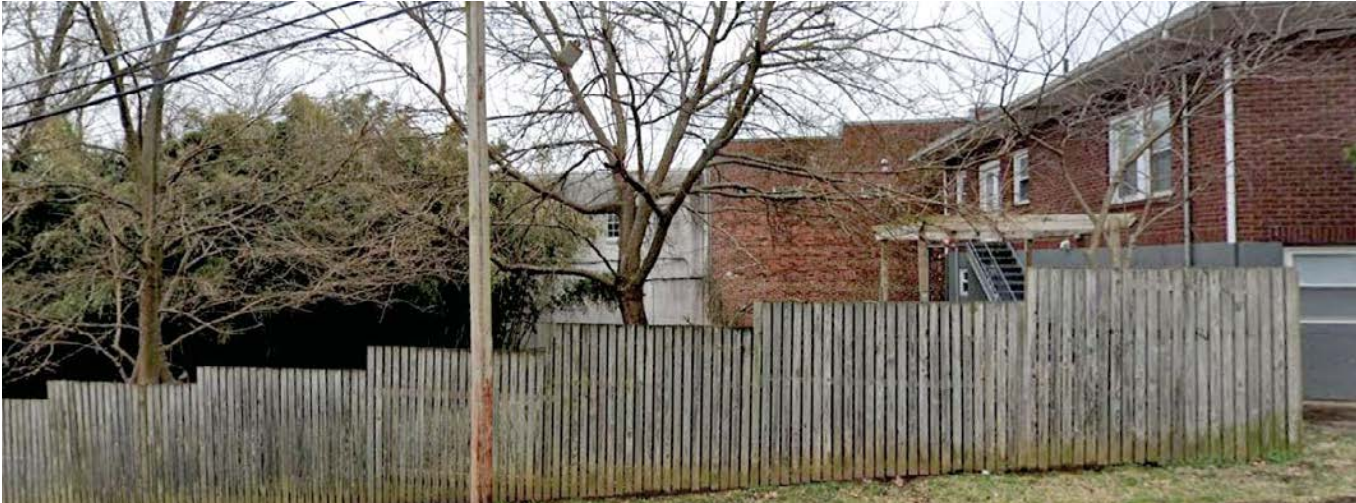
East Elevation from Harvey St, Neighboring Property in foreground. Vegetation and fencing obscure the view of the east side of the property.
