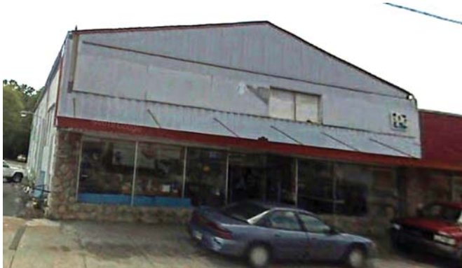
1121 N Central St | 2007 and 2019 (aluminum storefront, metal awning)
