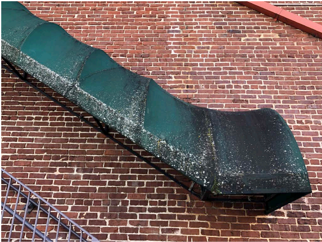
EXISTING FIRE ESCAPE STAIRS CANOPY
