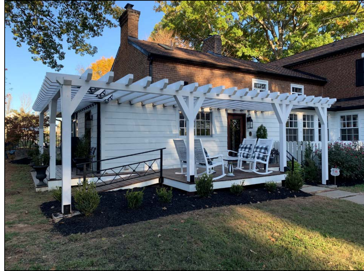
Additional views of pergola and deck
