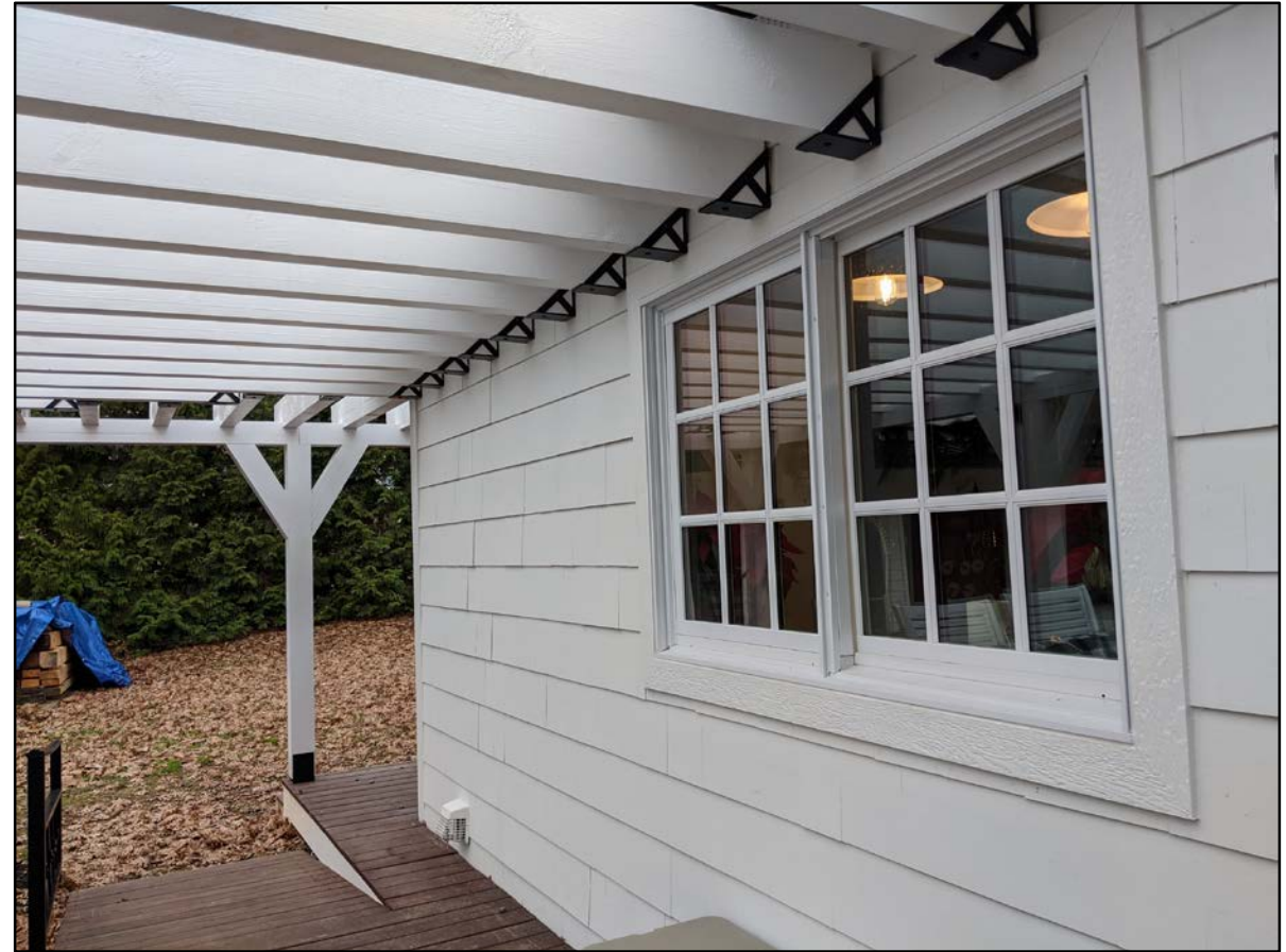
Window added to enclosed porch section
