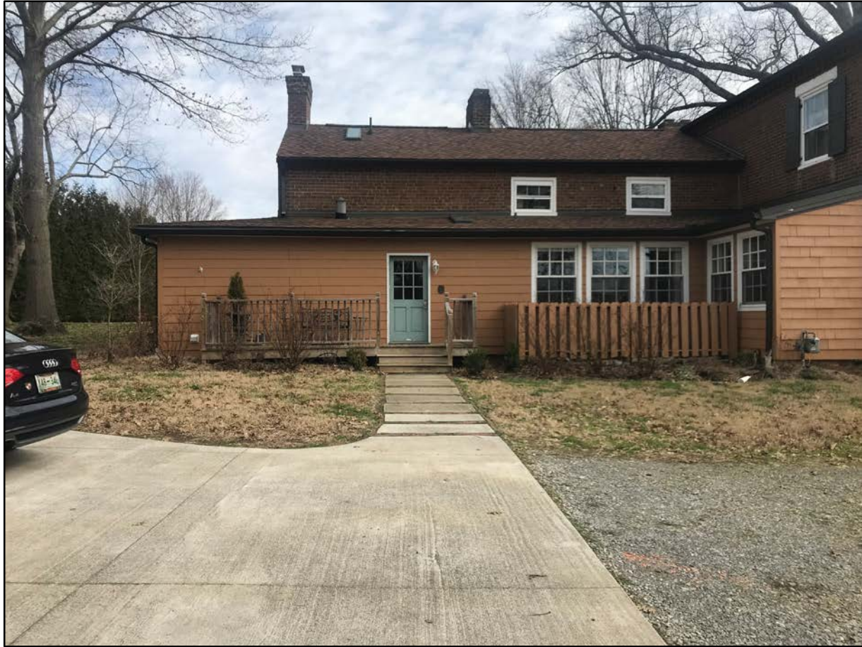
West elevation prior to work
