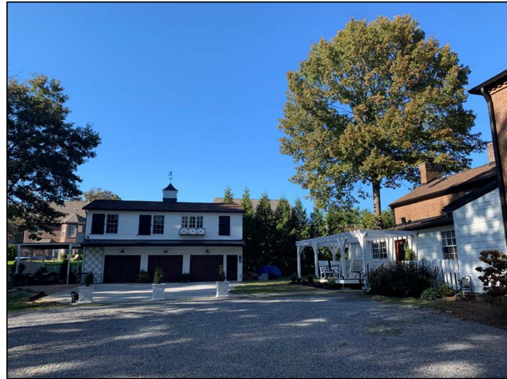
Carriage house as completed; depicting replacement garage doors, replacement door, replacement windows, and addition of cupola
