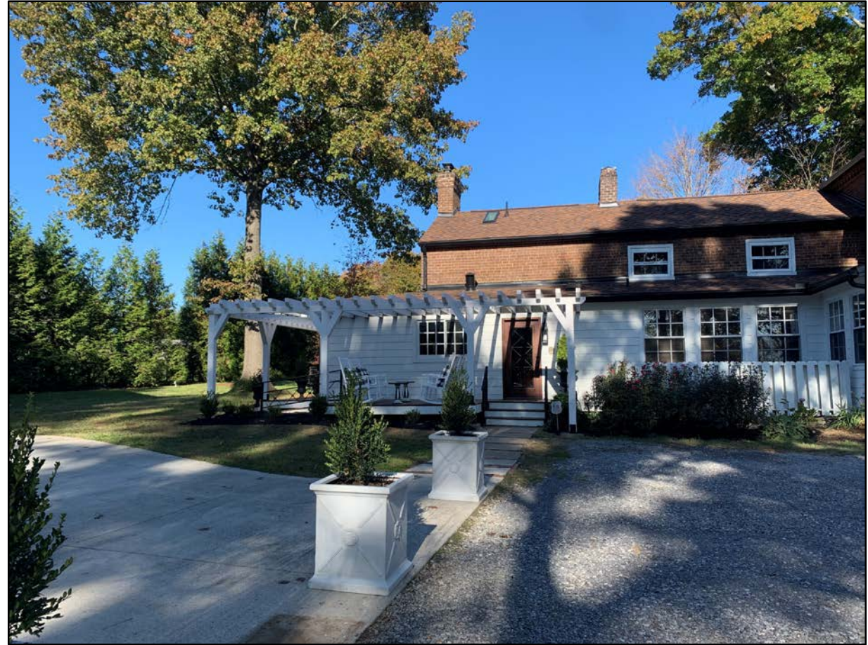
West elevation after work; pergola added to enclosed porch section, replacement door, one window added
