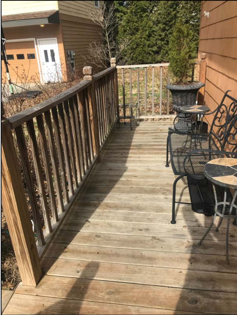
Views of deck before modifications
