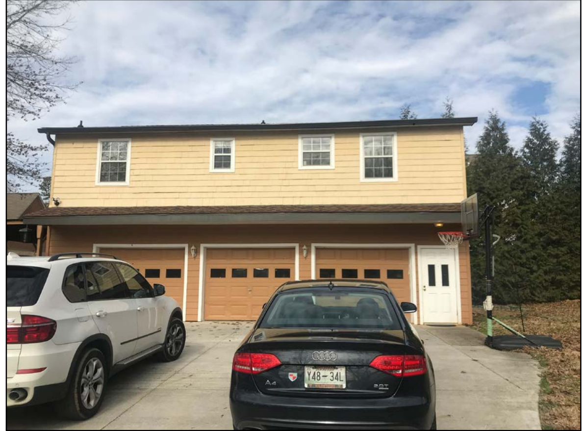
Carriage house, c. 1960, showing work completed in ~1990s
