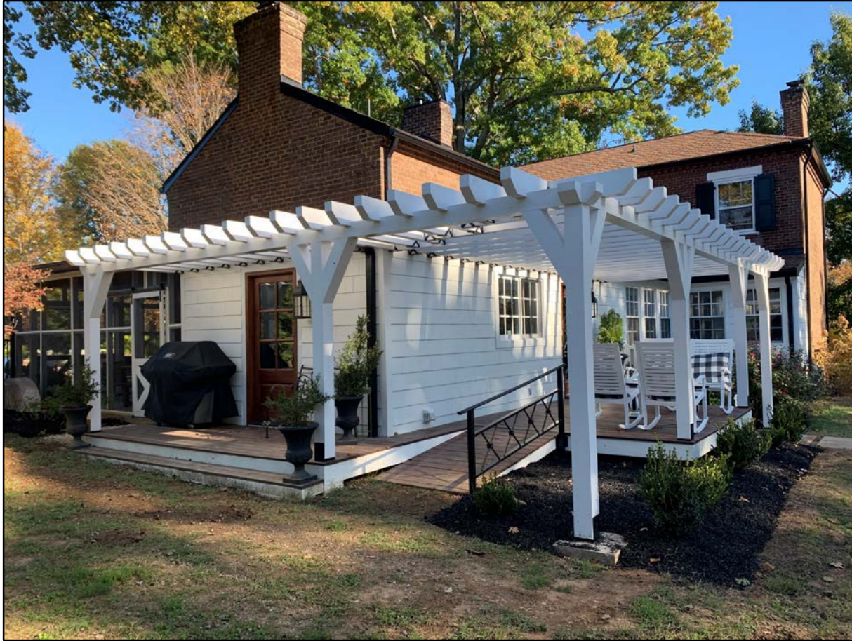
View of north elevation, pergola, and replacement door
