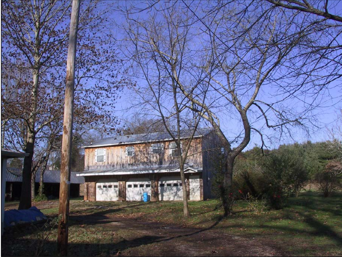
Carriage house, c.1960 Non-contributing to HZ overlay
