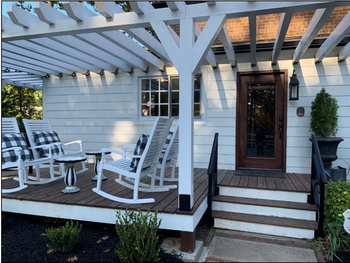
View of new window, deck, and replacement door
