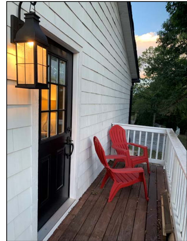
Additional door added on side elevation of carriage house
