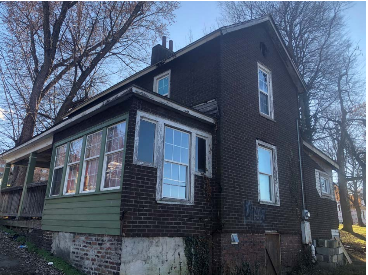
115 James Agee Street, photographer facing south
