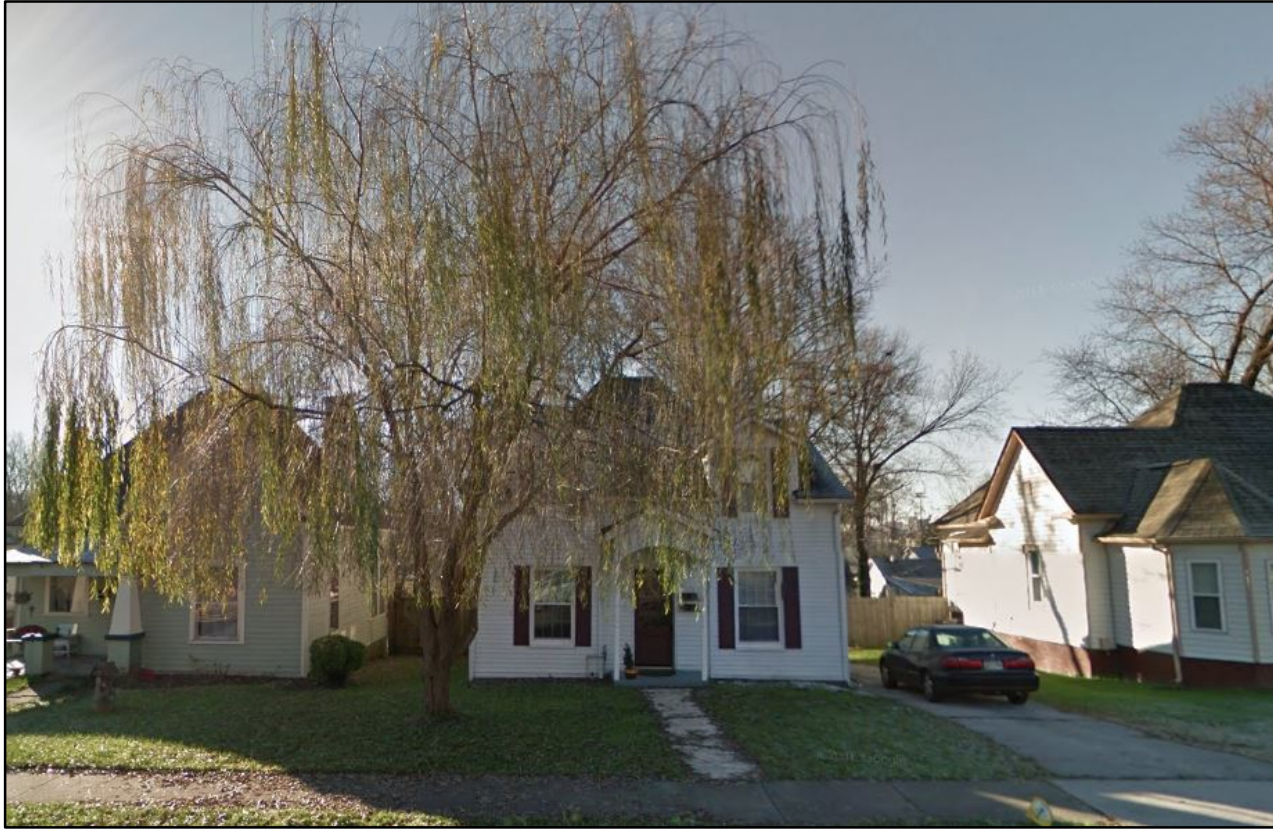
Façade, facing south
