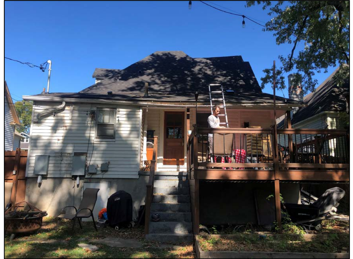
Rear elevation to receive solar panels, facing north
