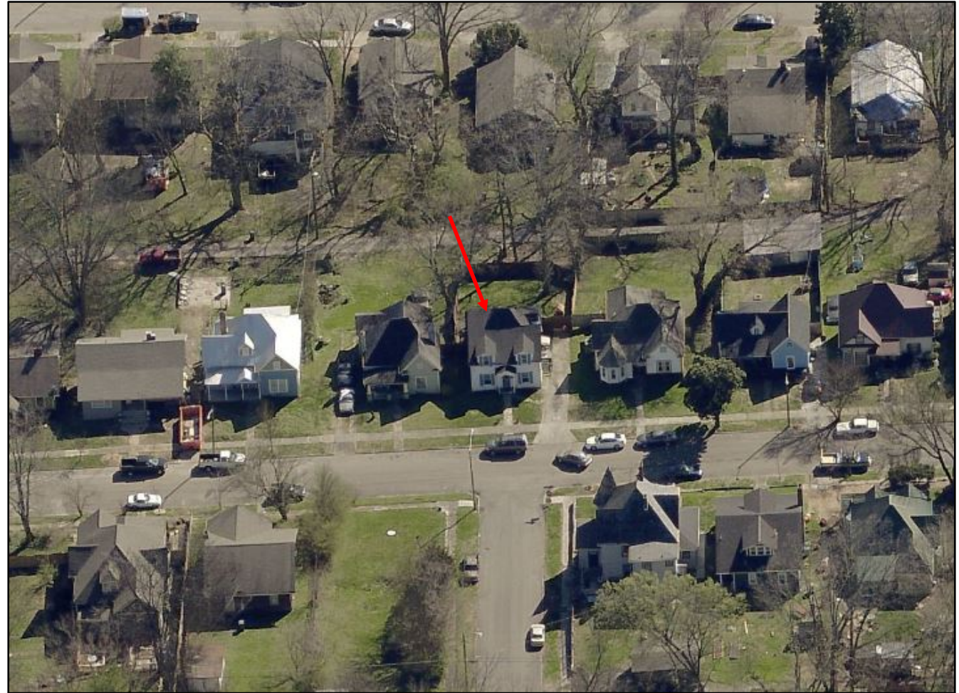
2018 aerial of property from Pictometry, facing south
