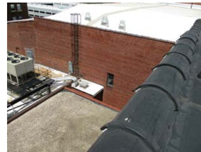
WEST ELEVATION FROM 612 ROOF
