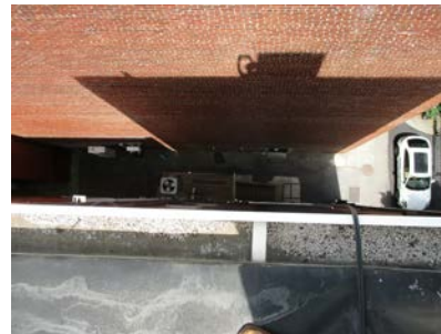
WEST ELEVATION LOOKING DOWN FROM 612 ROOF
