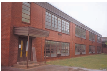
Before Window Replacement
