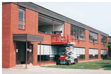
During Window Replacement
