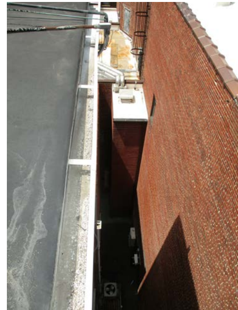
WEST ELEVATION LOOKING NORTH FROM 612 ROOF
