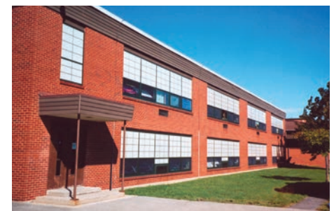
After Window Replacement
