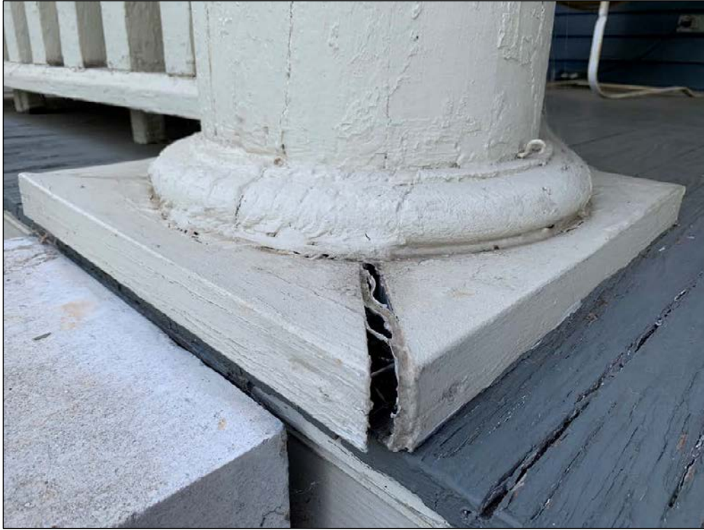
Porch column deterioration
