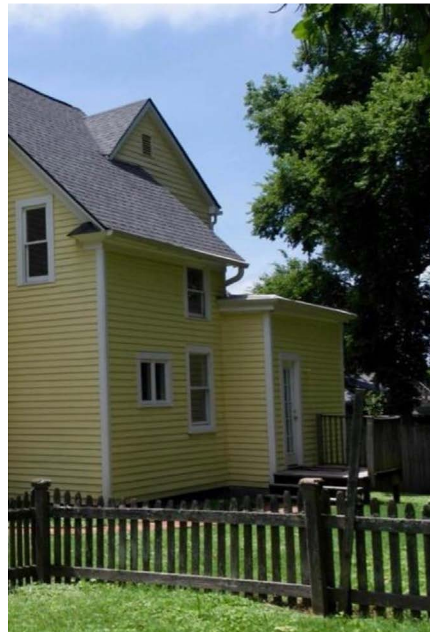
Previous deck on rear elevation
