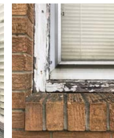
(Left to Right) Concrete stoop, likely mid-20th c.; Brick masonry porch foundation, likely original though concealed by brick veneer, likely mid 20th c.; Double hung windows, partly original, partly replaced, clad, or altered with storm windows, metal or plastic sills, etc.
