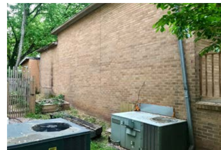
SIDEYARD ELEVATION Existing conditions
