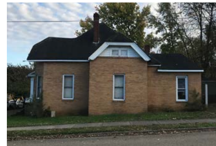
SECONDARY ELEVATION 3rd Avenue - Existing conditions
