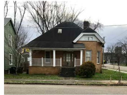
PRIMARY ELEVATION Luttrell Street - Existing conditions
