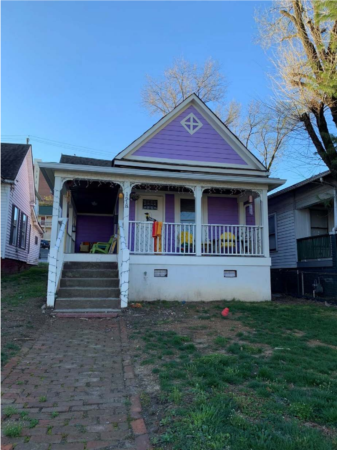
1618 Forest Front porch: (1616 will be identical when completed)
