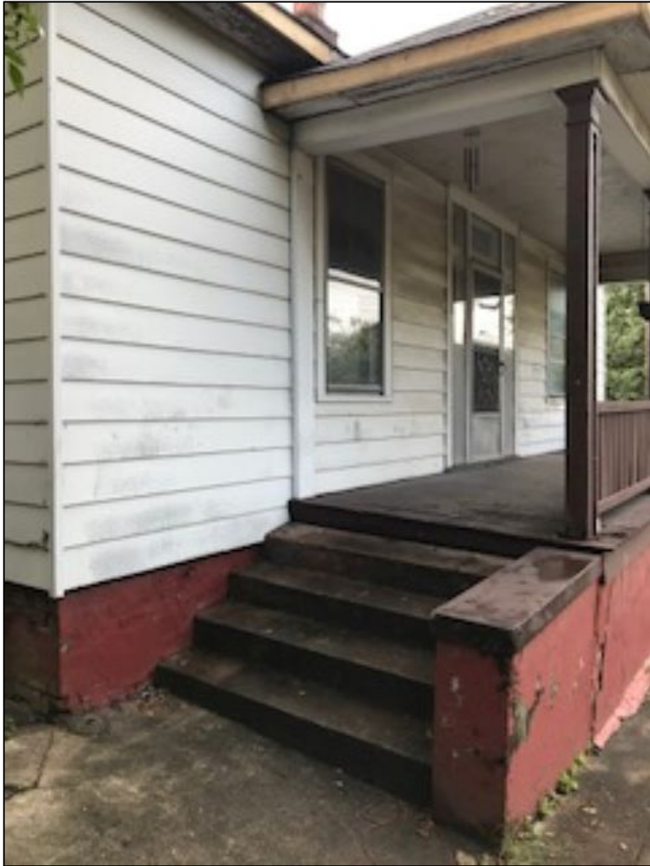
Existing porch steps, left side
