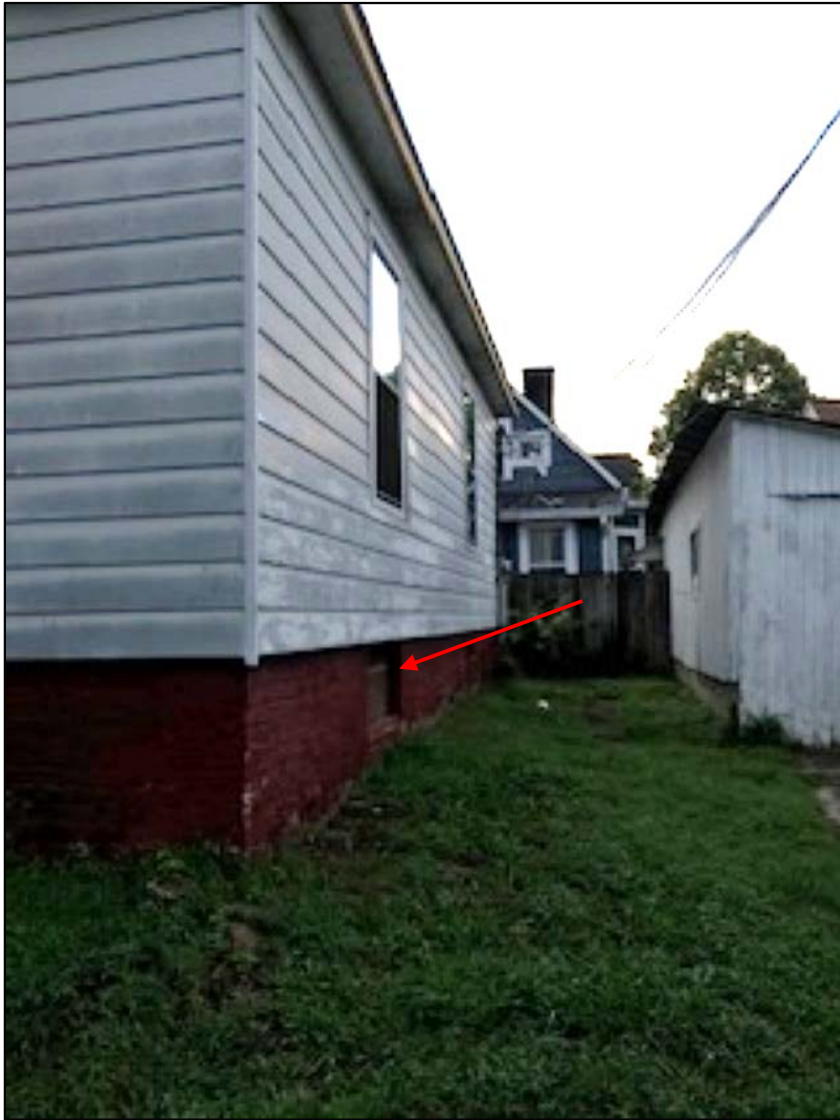
South elevation, photographer facing east
