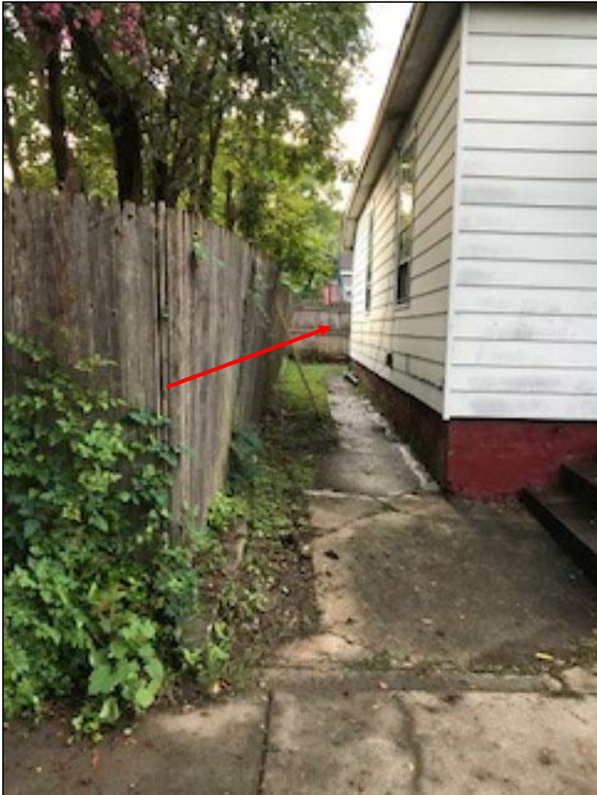
North side of house, photographer facing east
