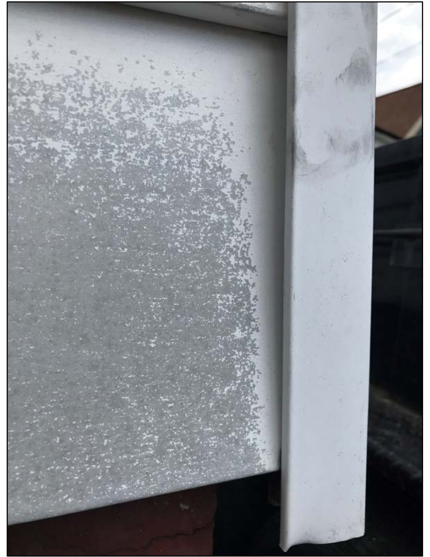
Existing aluminum siding
