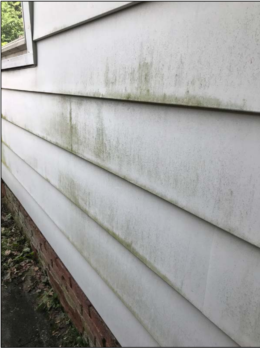
Existing aluminum siding
