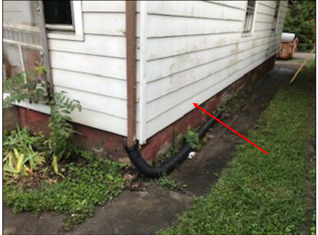
Proposed location of HVAC unit
