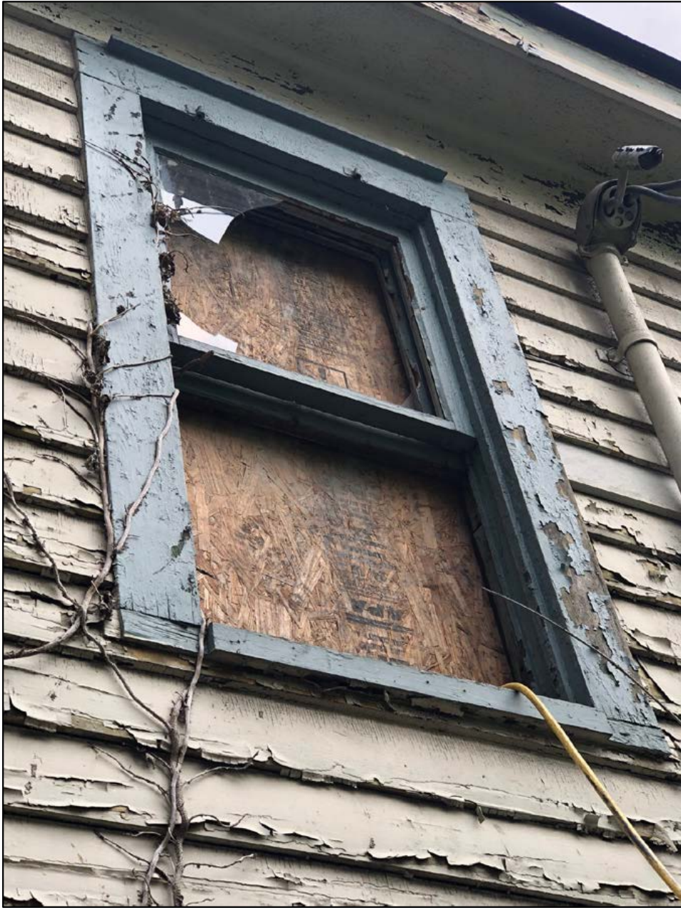
Evidence of deterioration of existing windows
