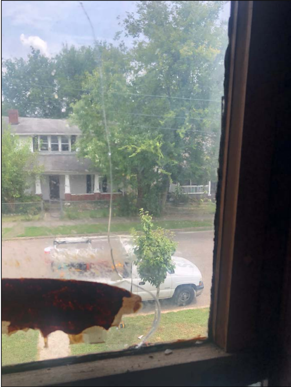
Evidence of deterioration of existing windows
