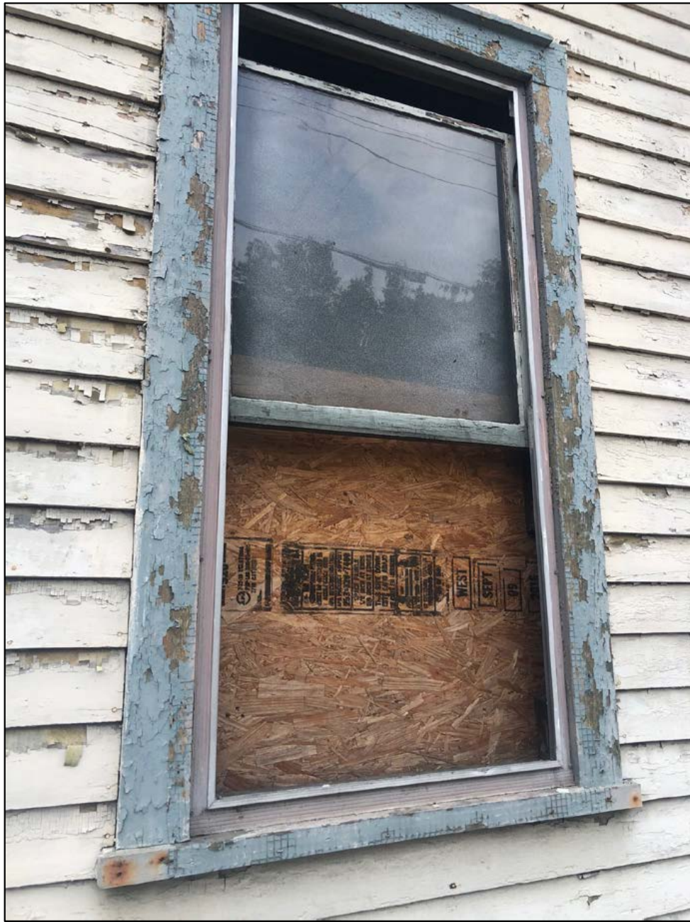
Evidence of deterioration of existing windows
