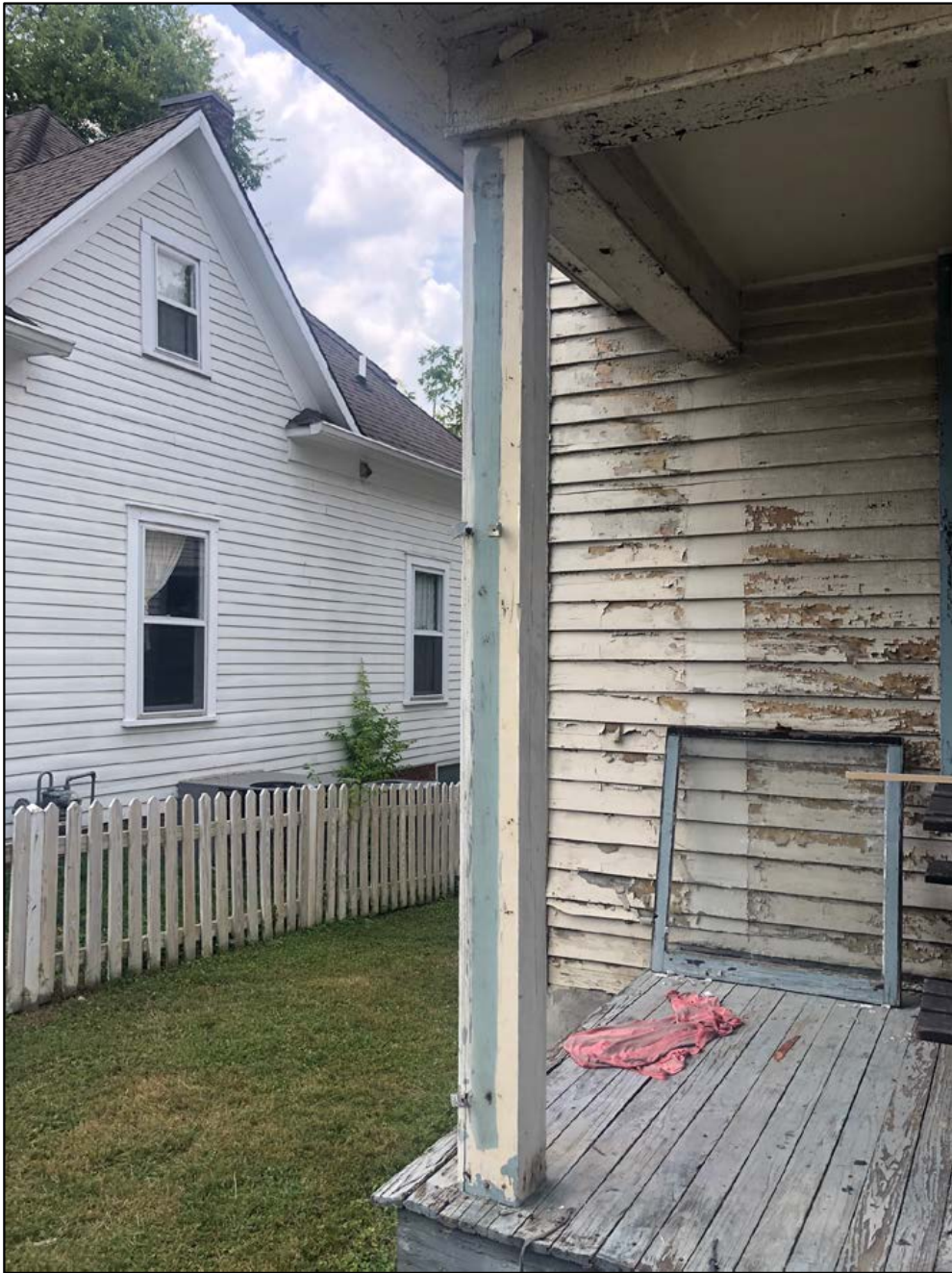
Existing porch columns
