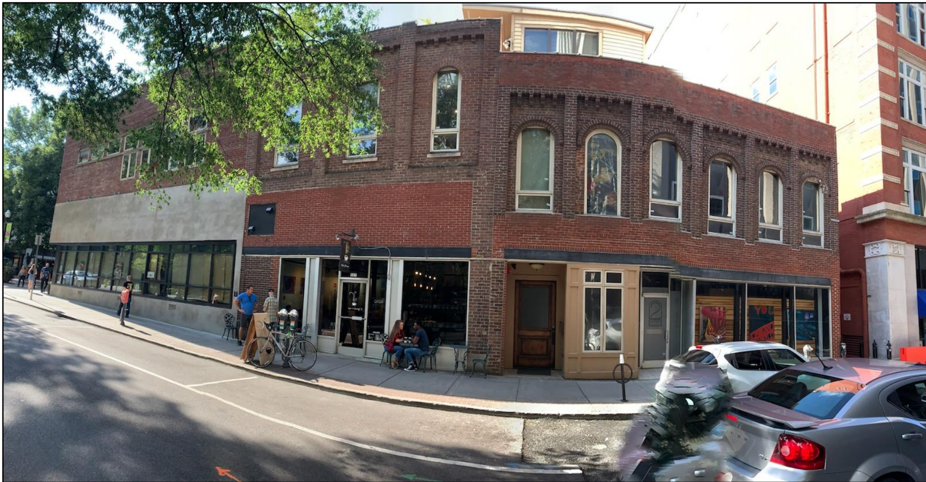
Union Avenue elevation showing extent of windows proposed for replacement (image distorted to show full elevation)
