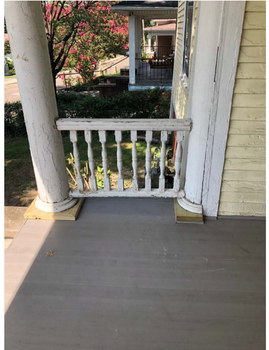
Square wood bases were replaced in-kind
