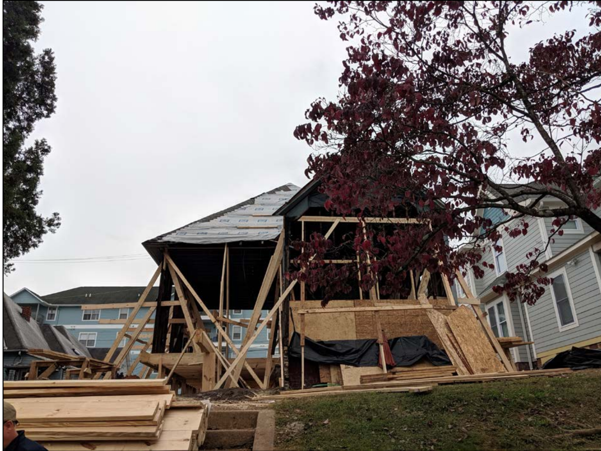
Façade (north elevation)
