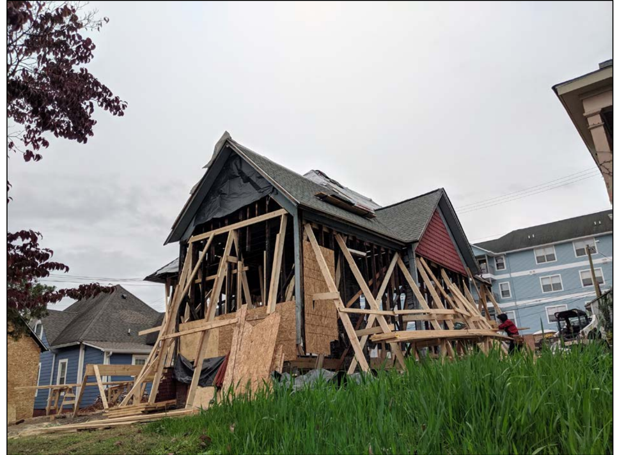
Northwest oblique view
