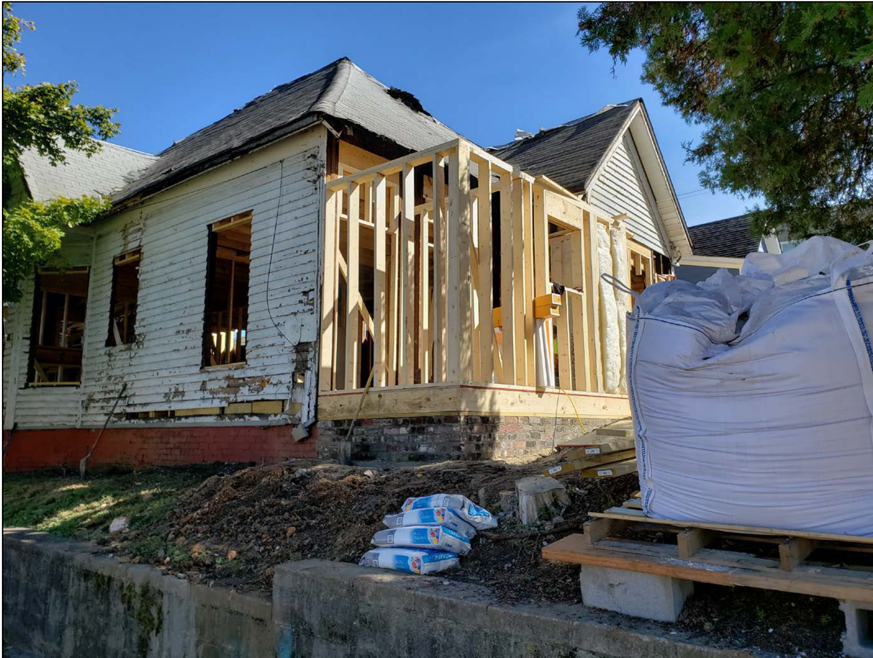
Rear elevation showing addition in progress
