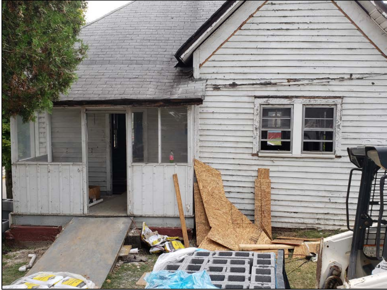
Rear elevation showing sunporch
