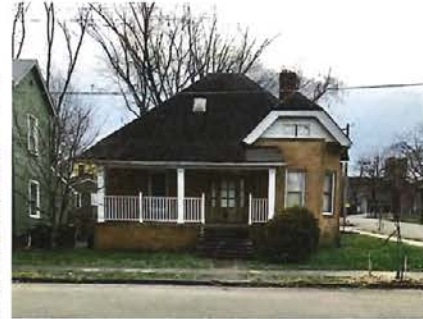
PRIMARY ELEVATION Luttrell Street - Existing conditions
