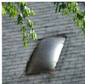
ASPHALT SHINGLE & YELLOWED SKYLIGHTS, CURBLESS
