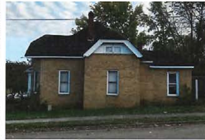
SECONDARY ELEVATION 3rd Avenue - Existing conditions
