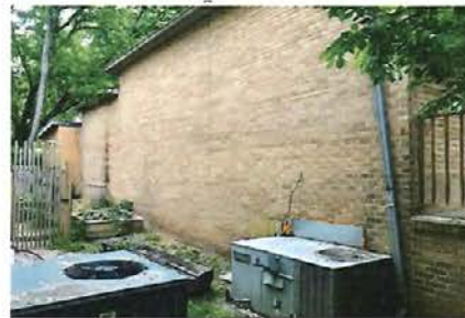
SIDEYARD ELEVATION Existing conditions
