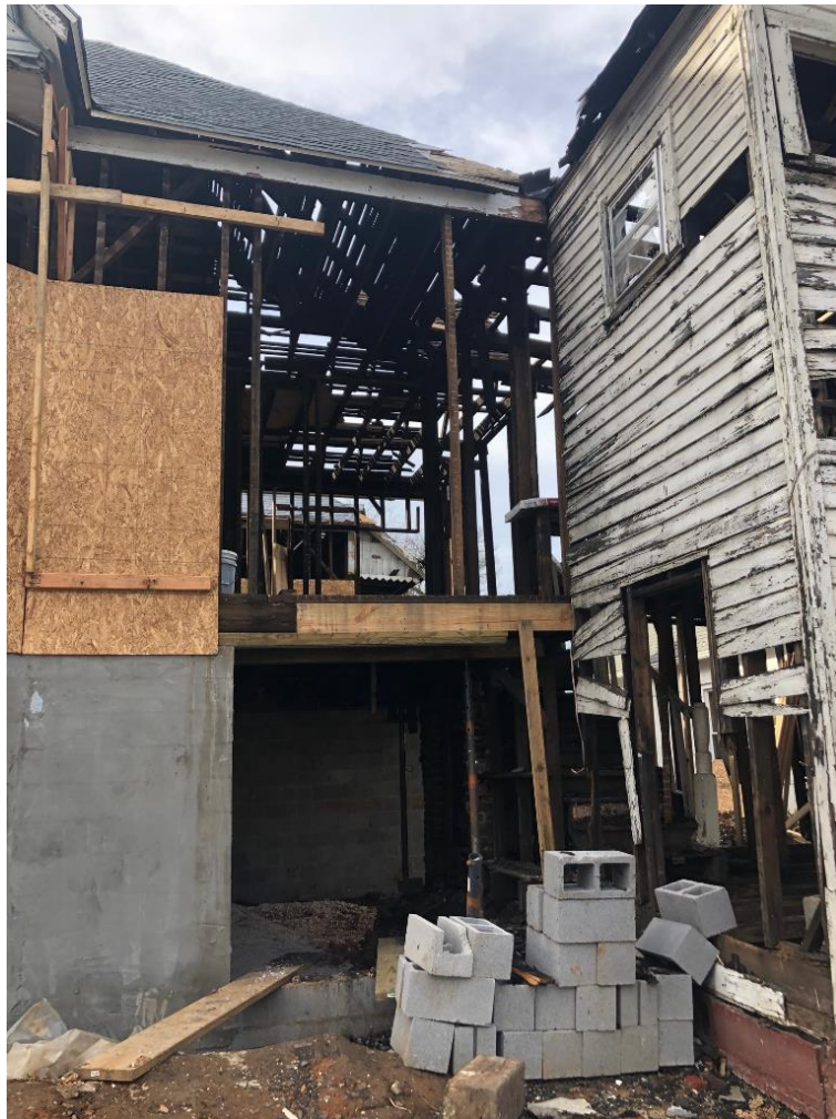
SIXTEENTH STREET SIDE BEFORE AND AFTER PARTIAL DEMOLITION
