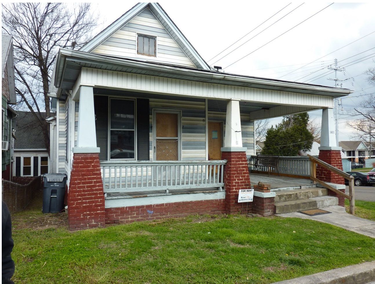
Front view facing south to Forest Av at corner of 16 th Street
