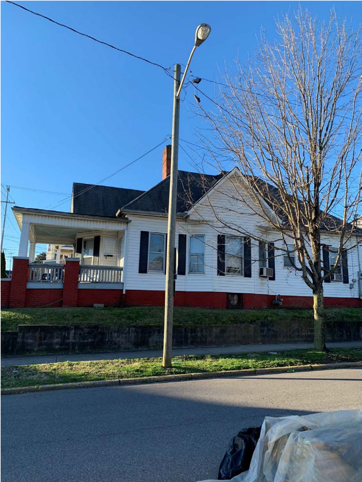
203 16 th (North) Egress window in place of attic vent. (36'x42" egress)
