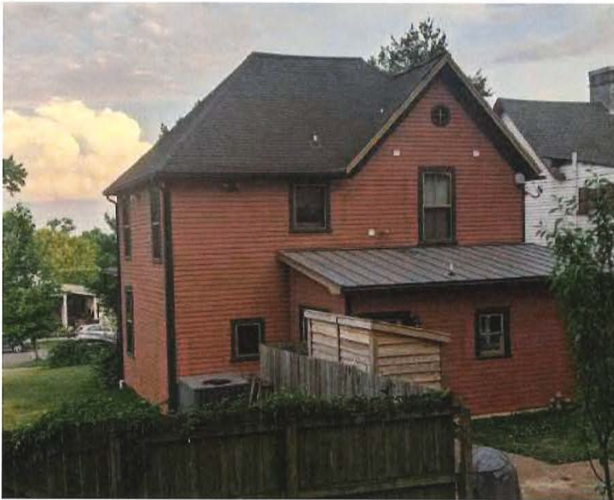
Rear angle view of home.
