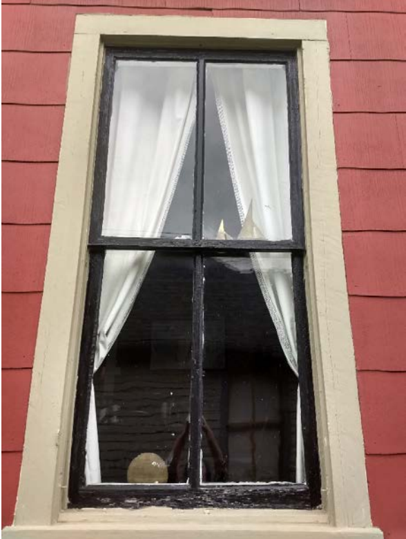
Images showing window configuration and condition of wood trim around windows.
