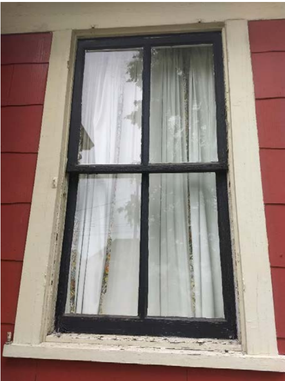
Images showing window configuration and condition of wood trim around windows.
