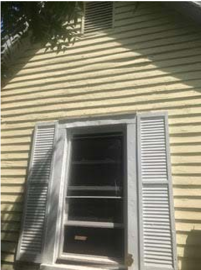
Photos of existing siding, submitted by contractor July 8, 2019
