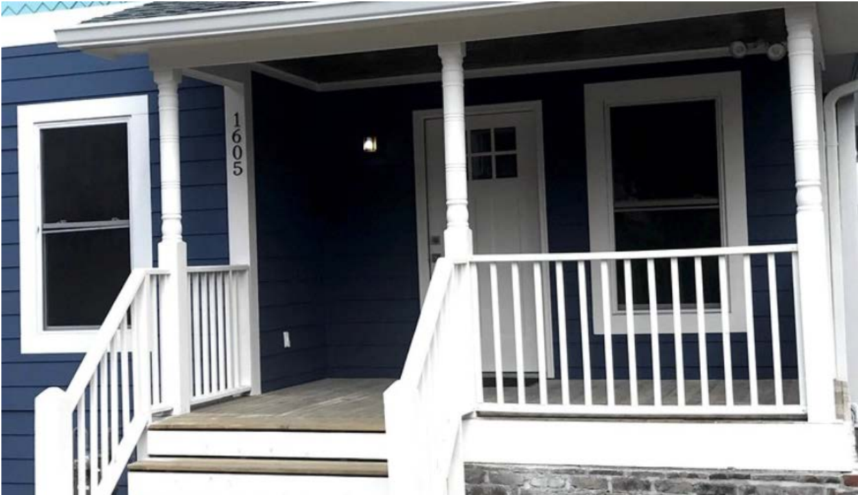
Railing Style & turned posts:
