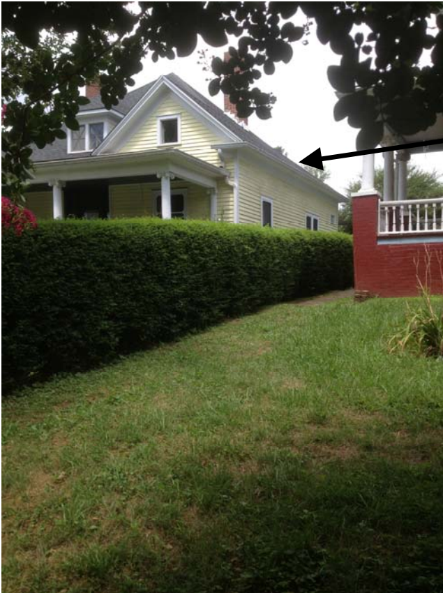
221 E. Oklahoma Ave – View of north side
