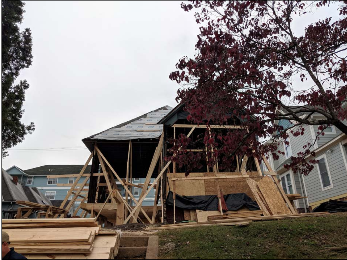
Façade (north elevation)
