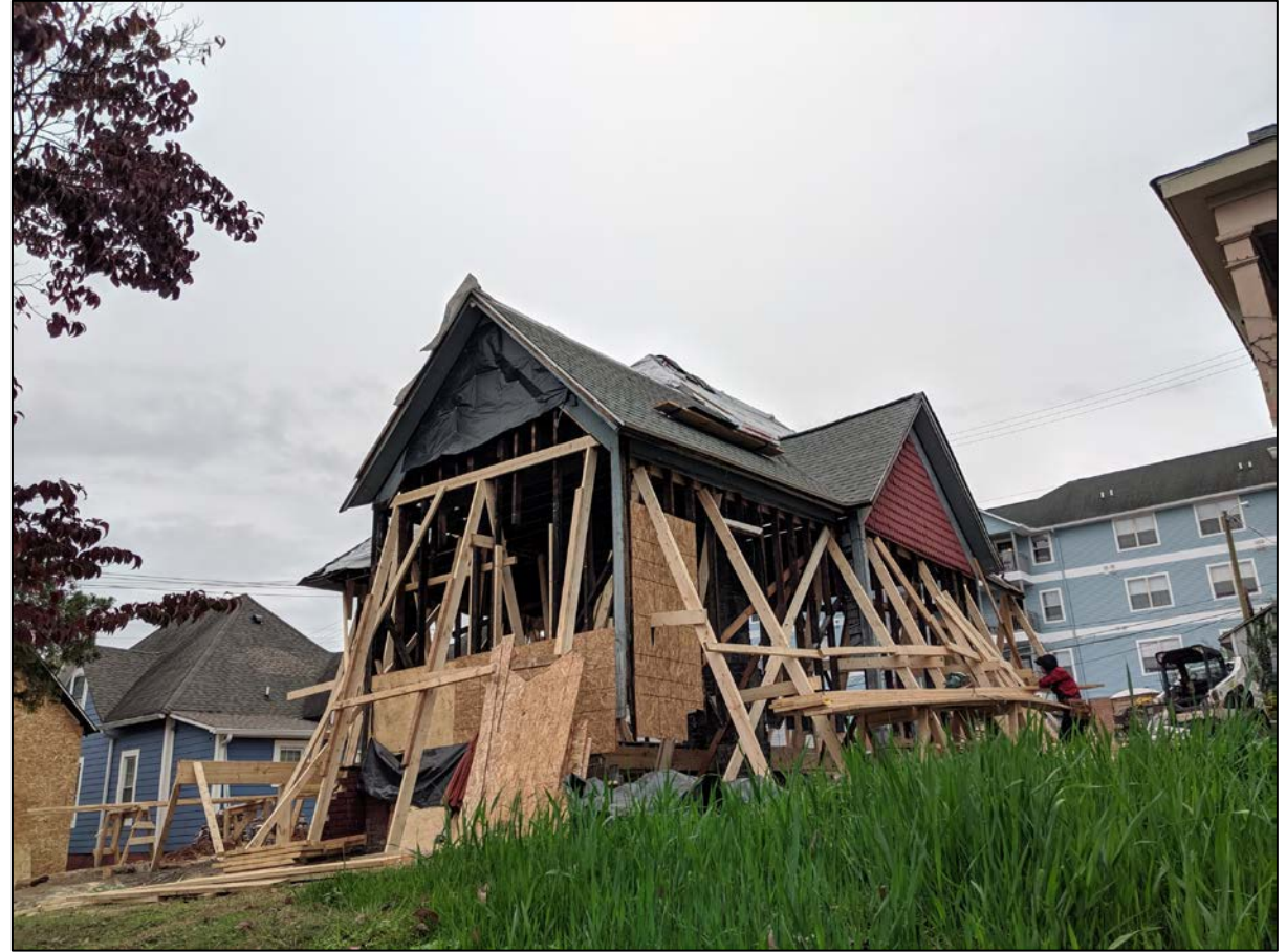
Northwest oblique view
