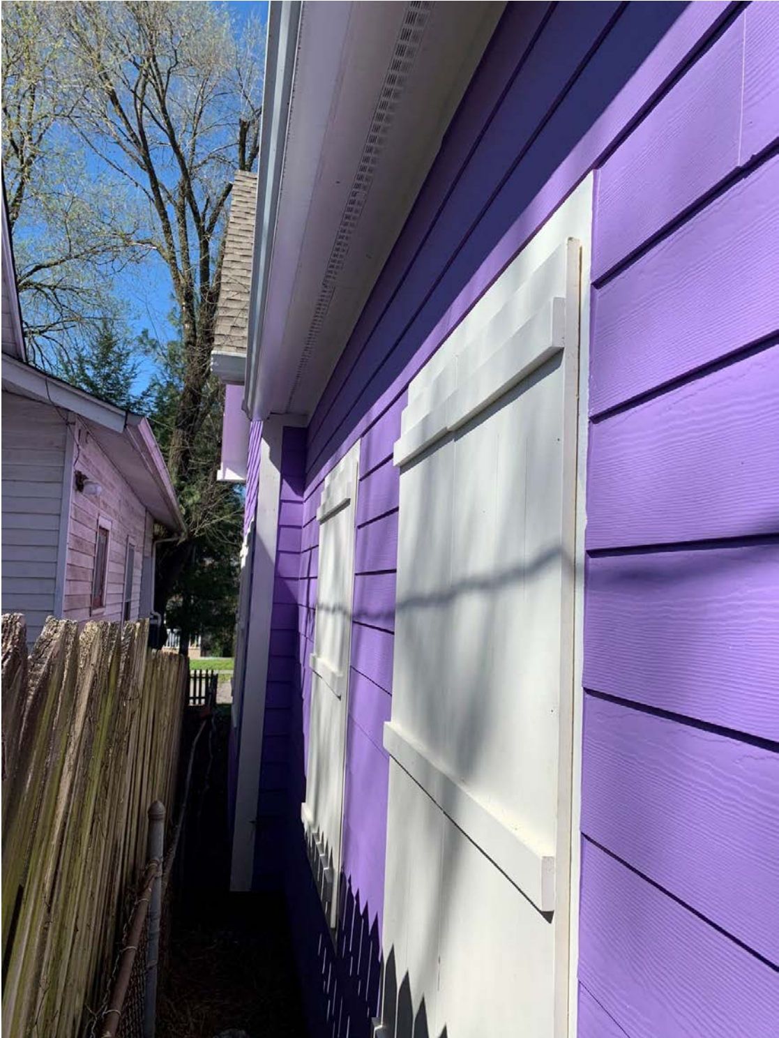
Window Covers Example on fire walls
