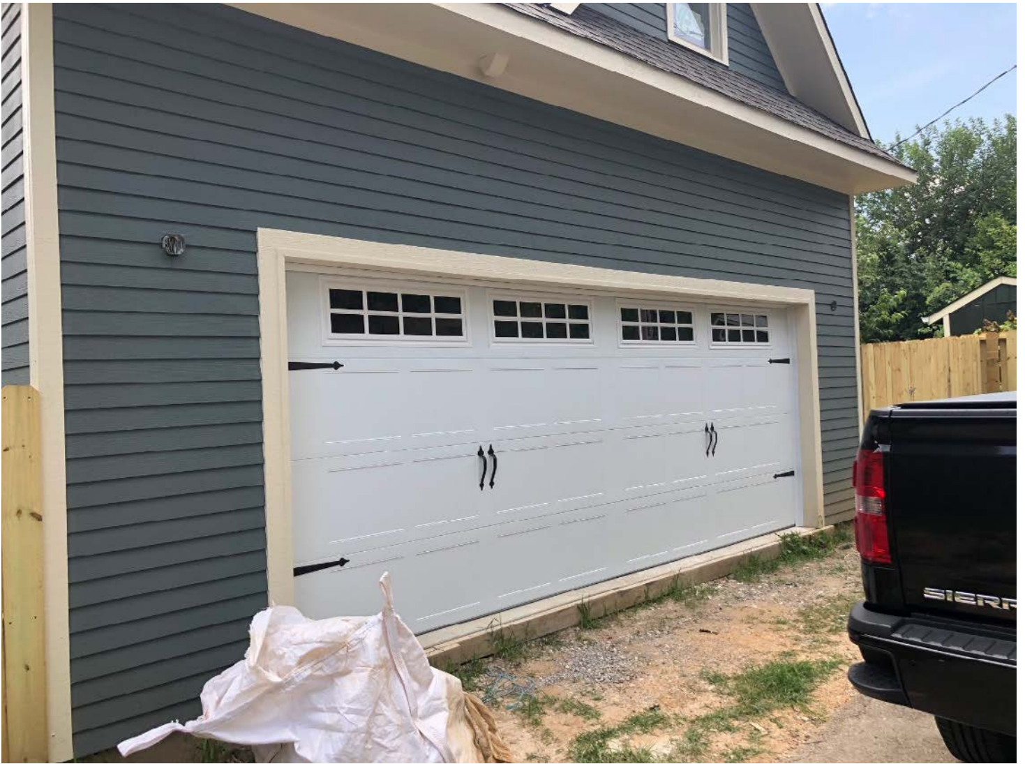
1019 Eleanor - New garage with faux-grained fiber cement board siding (photo provided by applicant)
