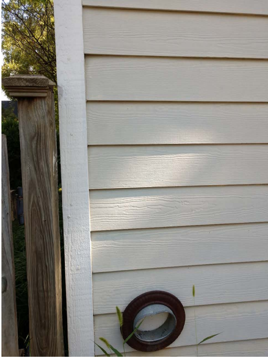
Faux-grained fiber cement board on early shed in Fourth & Gill H-1 Overlay –constructed in 2004
