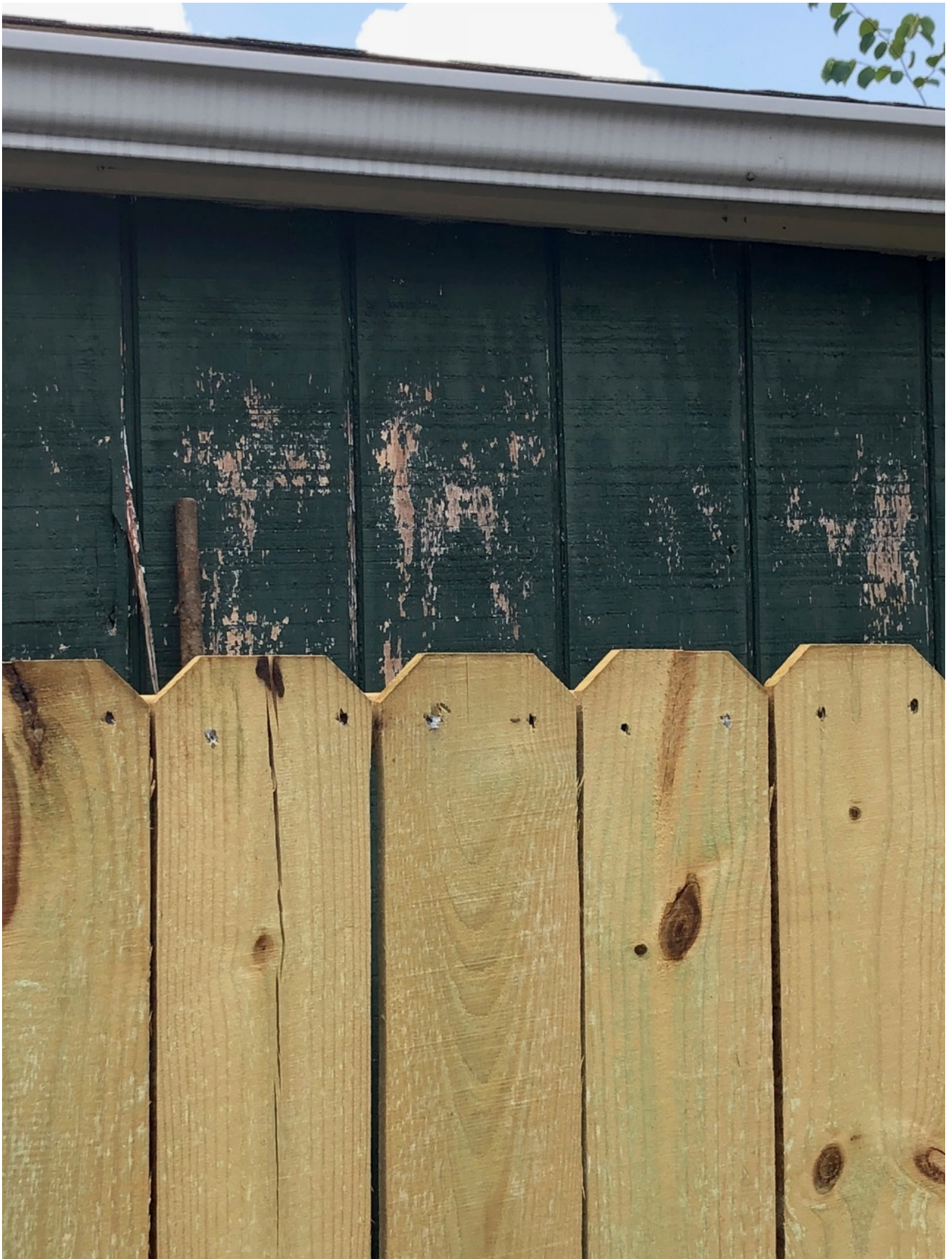
Example of rough-hewn cedar siding (photo provided by applicant)
