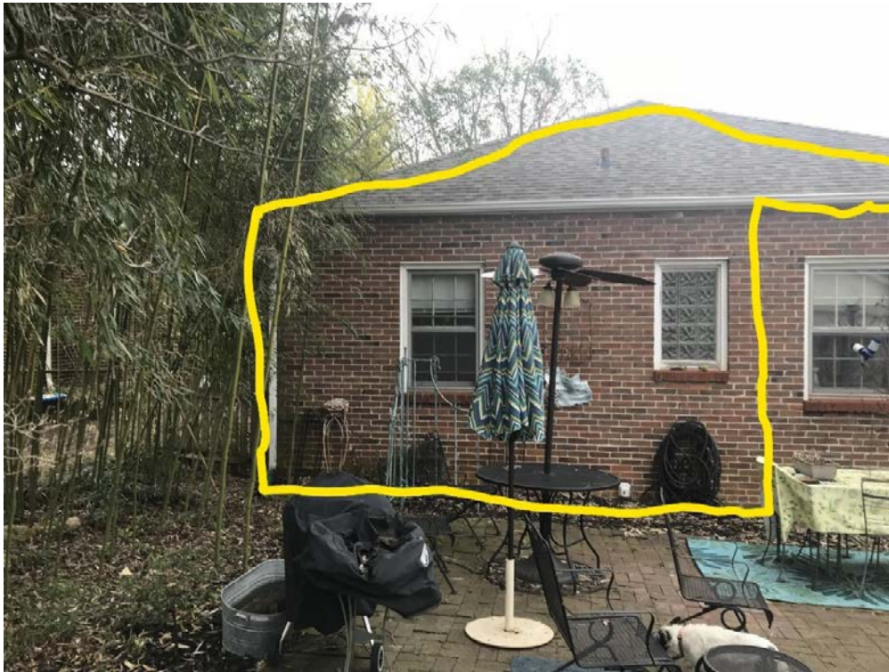
2212 Emoriland - Rear showing location of addition – West end
