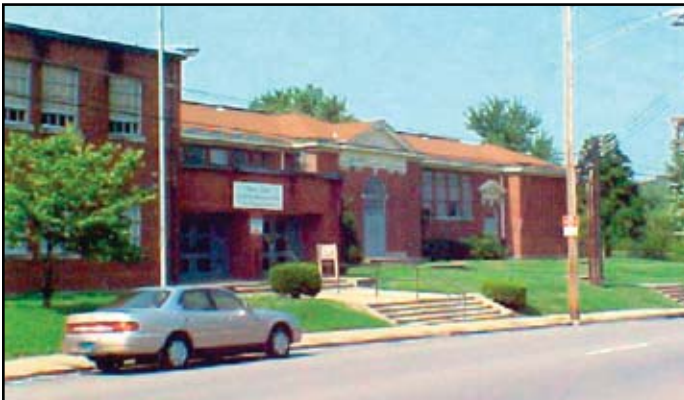
The school prior to rehabilitation.
