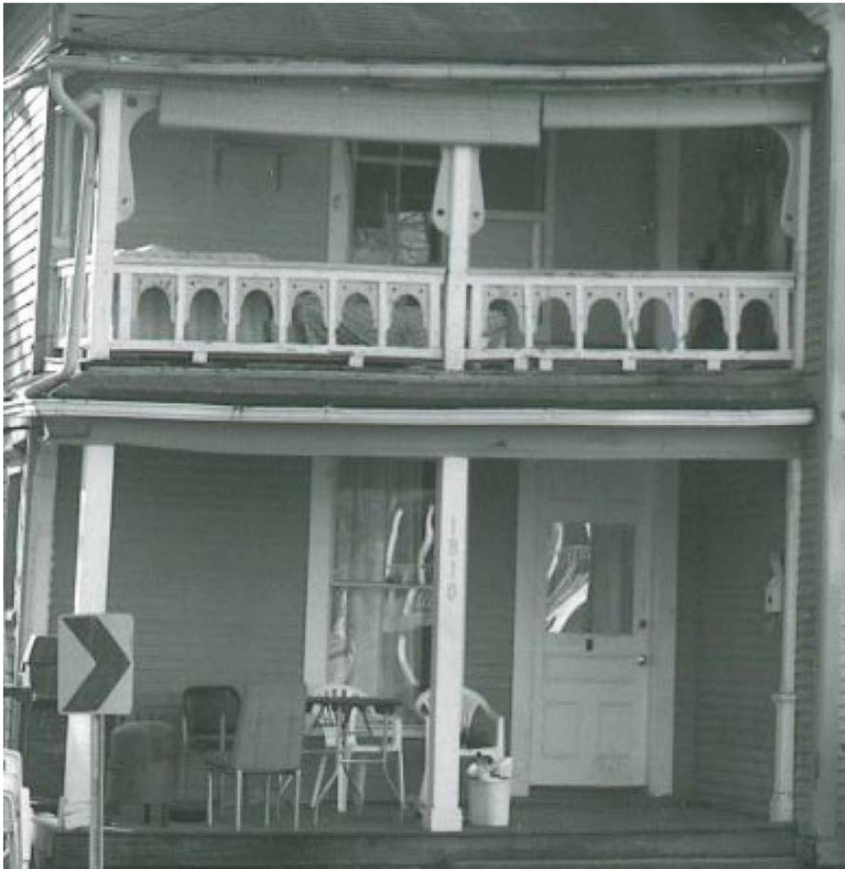
1810 Highland Avenue -- 1990 or 1996 survey -- sawnwork indicates George Barber influence
