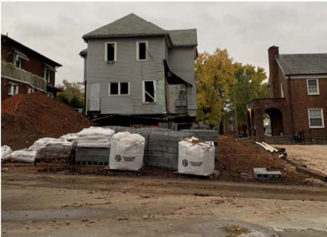
1717 Laurel Avenue as existing viewed from the rear alley
