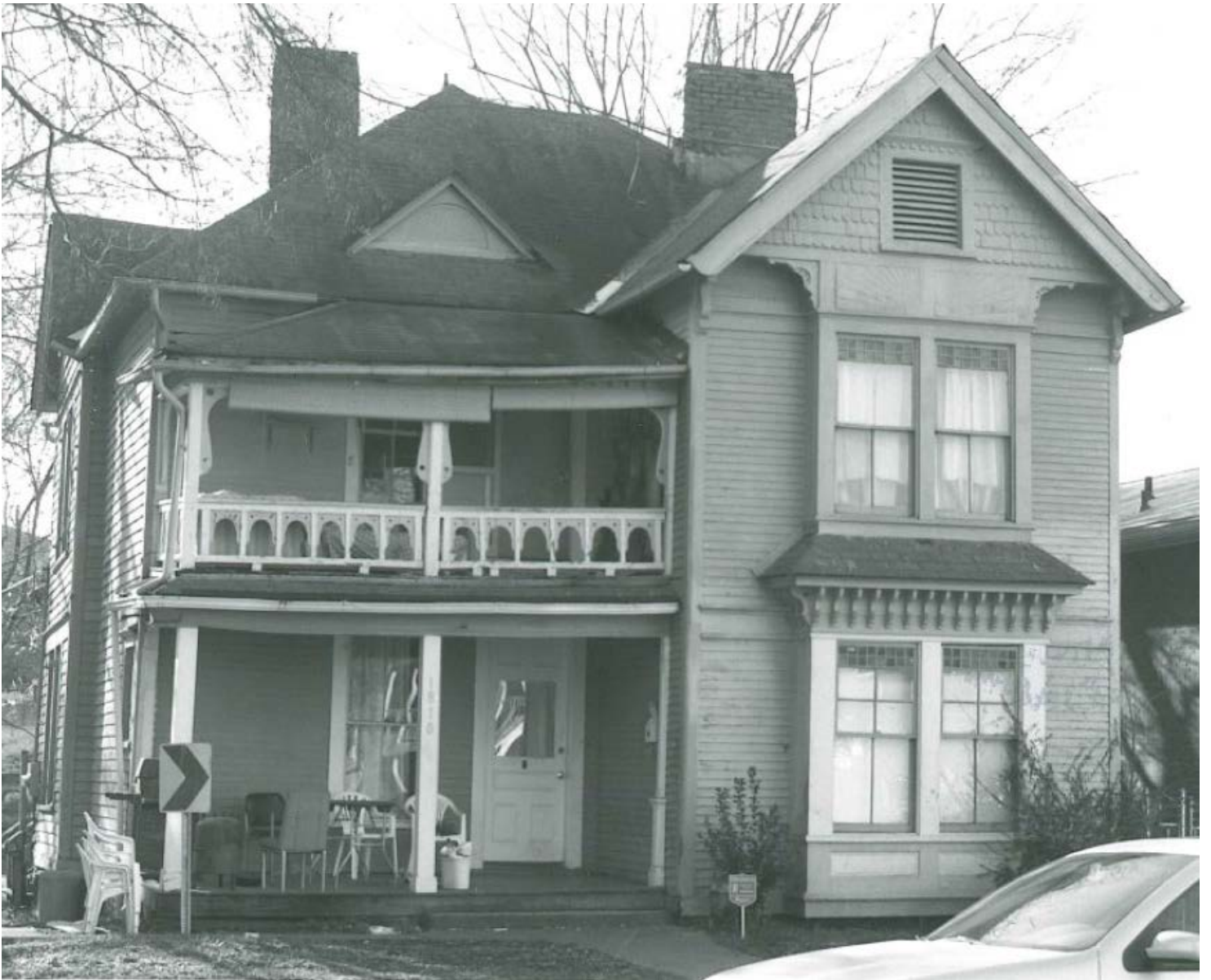
1810 Highland Avenue -- 1990 or 1996 survey – sawnwork indicates George Barber influence
