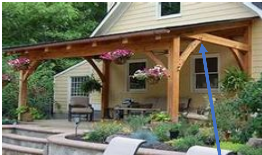
Example of simple wood beams and posts. Would not use curved braces.
