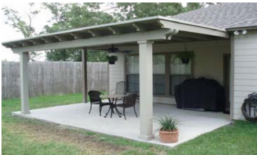
Example of painted wood beams and posts. Would not use decorative ends.
