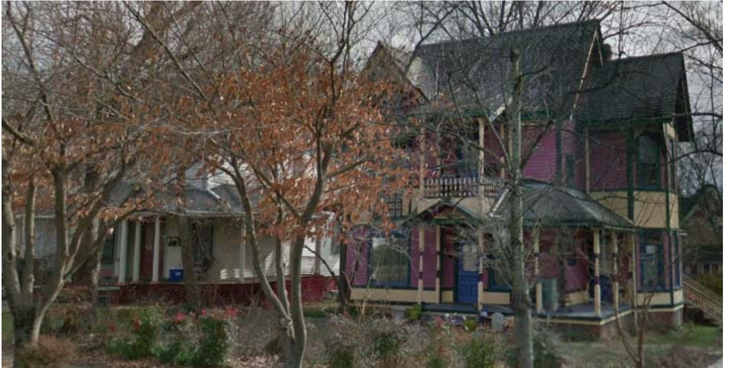
1704 Washington Avenue and 1702 Washington Avenue as viewed from the west
