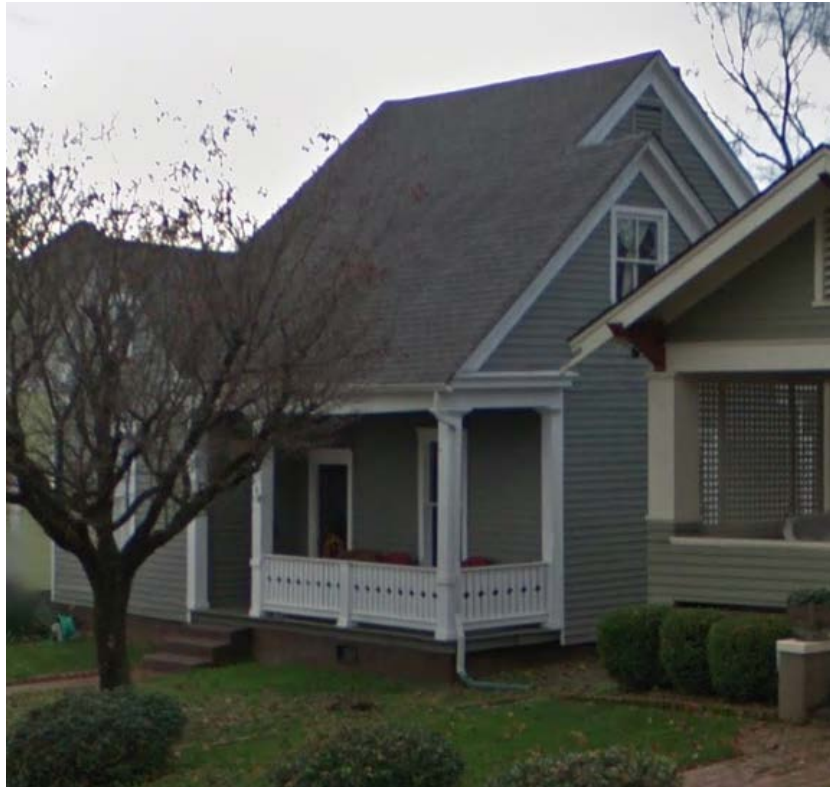
134 Grainger Avenue double-hung window added in lower side gable (ONK H-1 in 2013) Original rectangular attic vent retained in upper gable.
