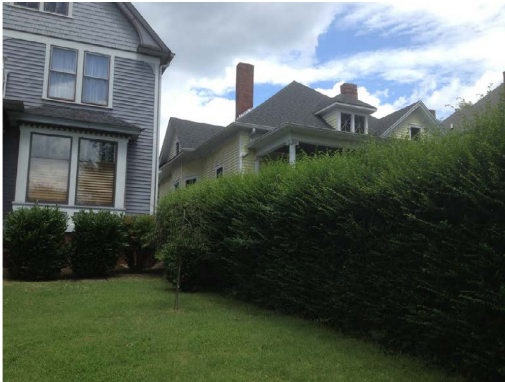
221 Oklahoma Avenue double-hung window approved on south side gable (ONK H-1 in 2012). Existing attic vent not original since there was an existing complete window frame and casing in the vent opening. The window was proposed to be installed on a side elevation that was not highly visible due to the setback and elevated topography.
