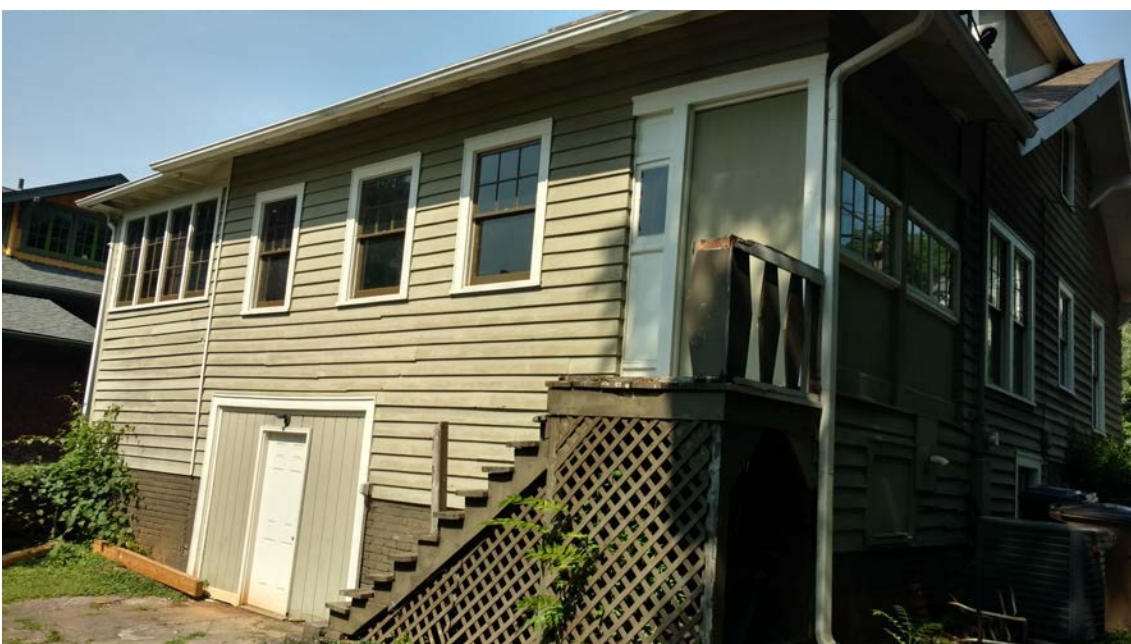
1318 Armstrong - Rear facade
