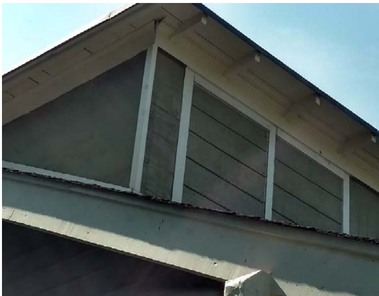
1318 Armstrong - Side and front of dormer showing siding
