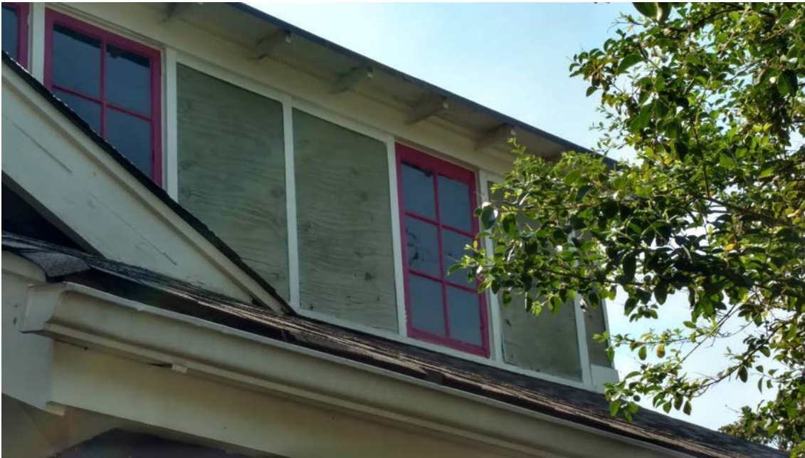
1318 Armstrong - Front dormer with existing plywood sheathing
