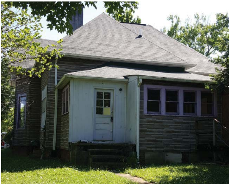
1437 Grainger Ave. rear façade (5/2018)
