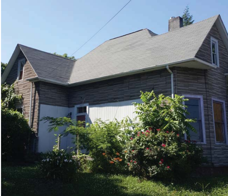
1437 Grainger Ave. front façade indicating missing porch (5/2018)
