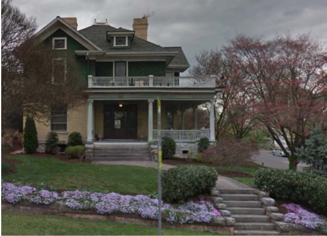
230 W. Glenwood Avenue—Front facade
