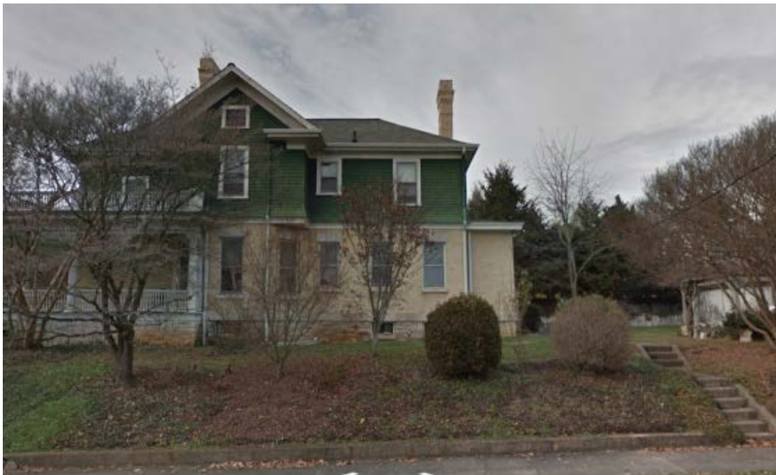
230 W. Glenwood Avenue—East side facade
