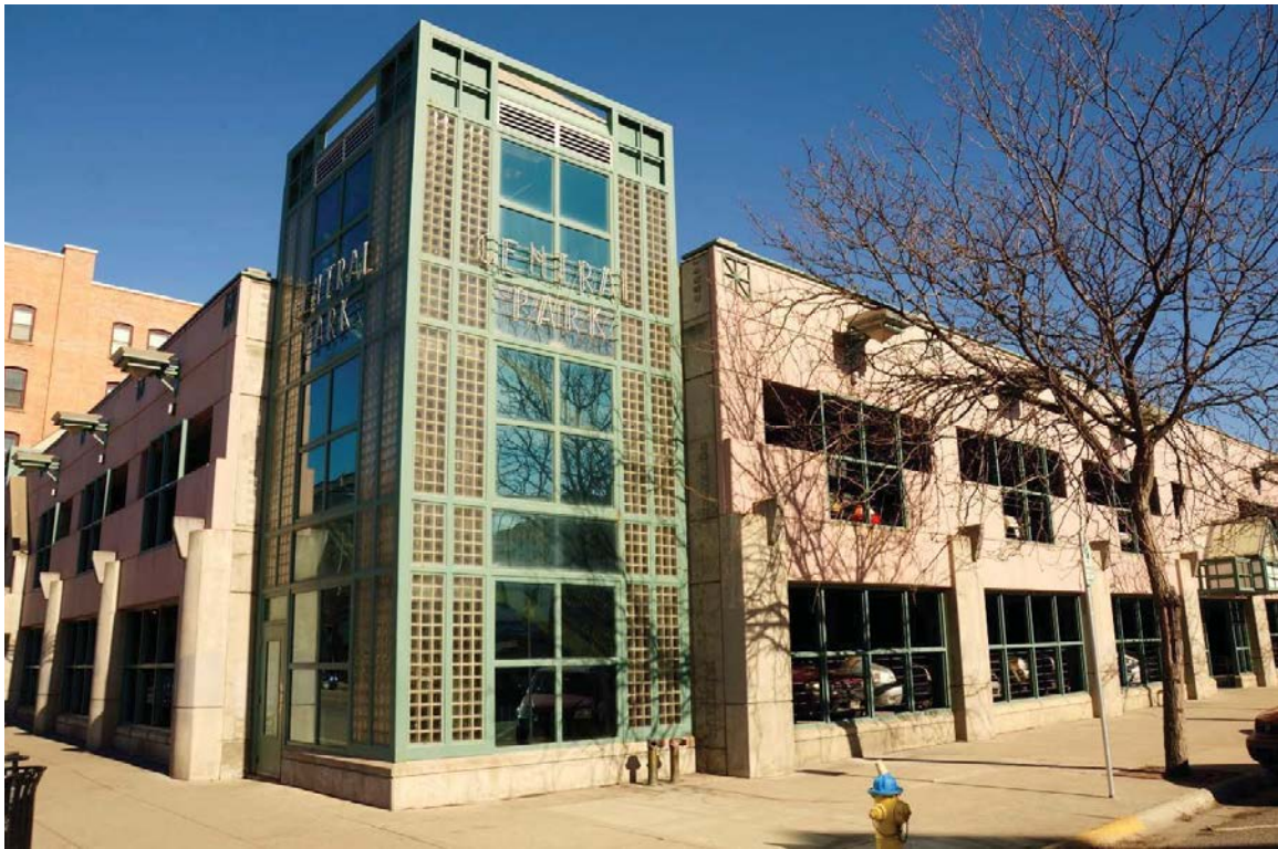
Parking garage examples showing bays with vertical articulation, and breakdown of openings to read as windows.
