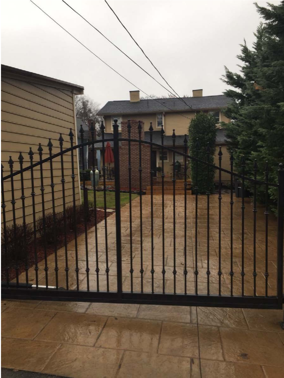
809 Eleanor - Rear view showing deck from alley
