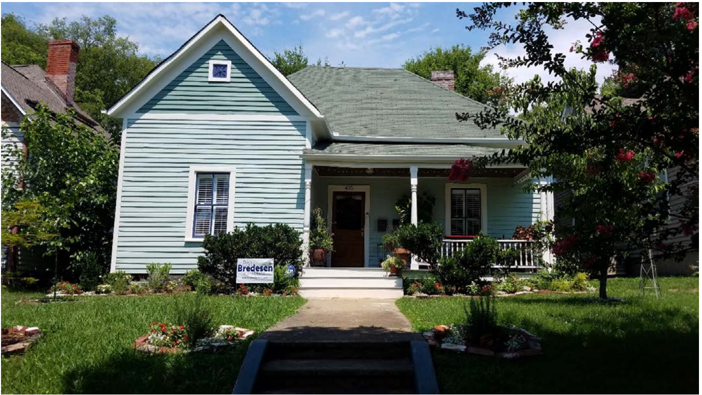
405 East Oklahoma – Front façade
